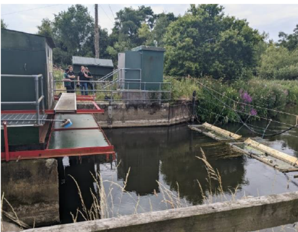
Photo 2: View of fish monitoring hut perched on central piers and telemetry hut
