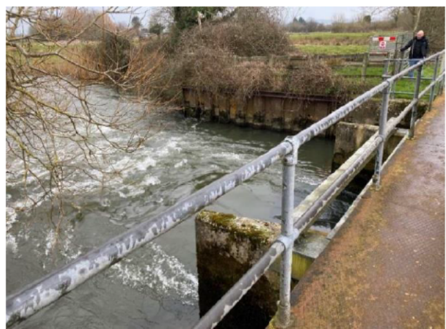
Photo 3: Central piers as viewed from flume structure footbridge
