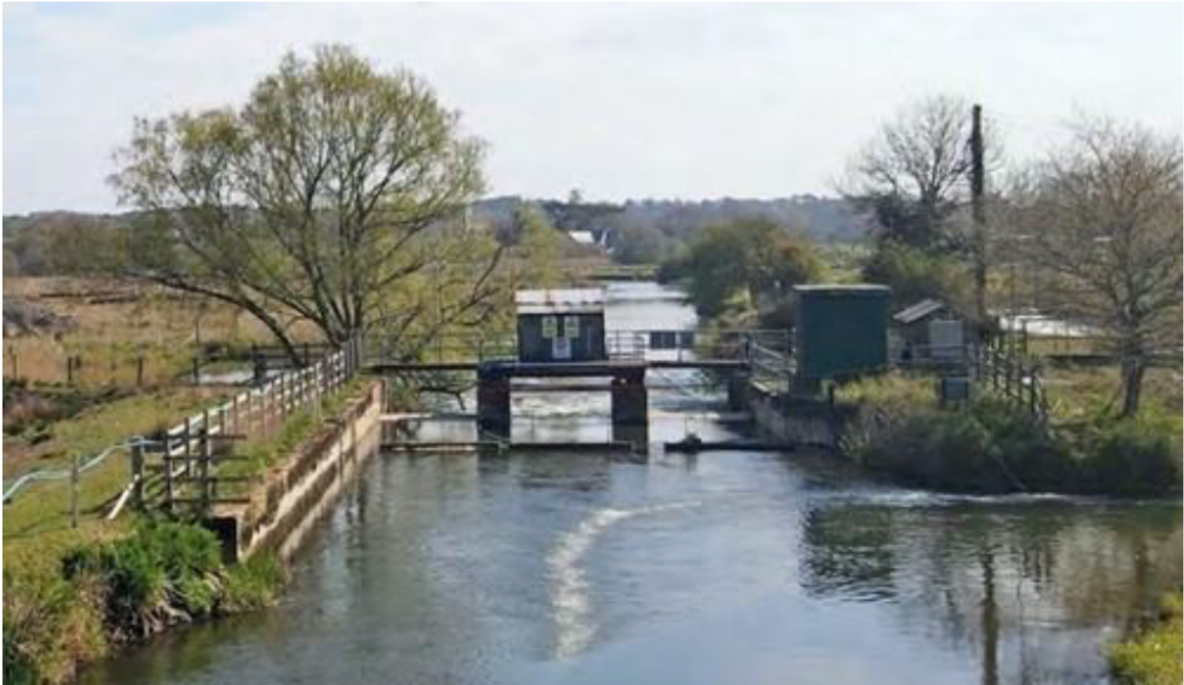
Photo 1: East Stoke Weir viewed from the upstream
