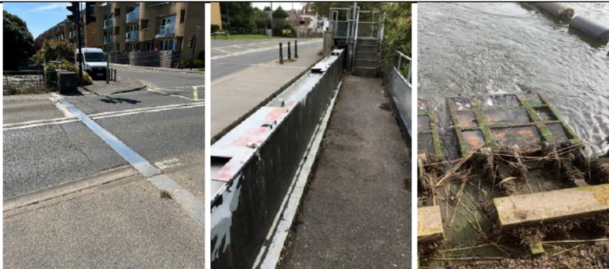
Photos – left to right. Sill, walkway behind the flood gate and tidal flaps.
