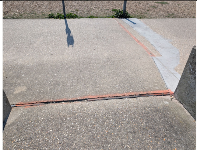
Photo 2: Red painted line depicts point of subsidence at a construction joint crossing the ramped entrance to the promenade
