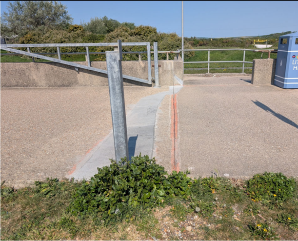
Photo 1: Red painted line depicts point of subsidence at a construction joint crossing the promenade
