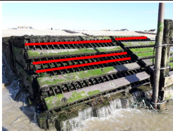
Photo 3. Front view of the security cage and baffles. Red lines indicate the missing baffles.
