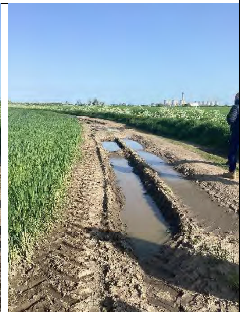
P3 – Damage to access track
