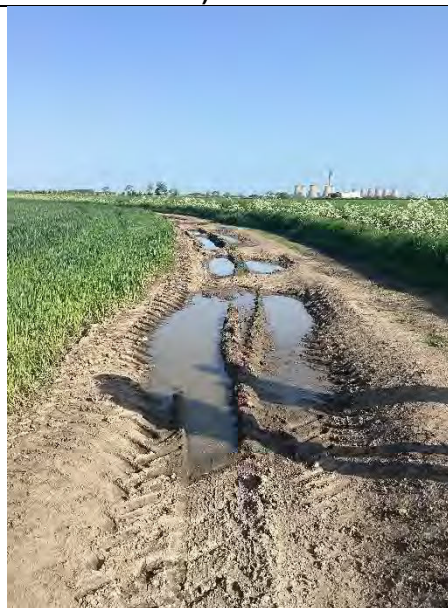
P2 – Damage to access track
