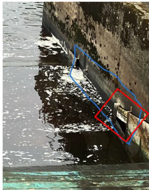
Photo 5: Missing and damaged panel boards
