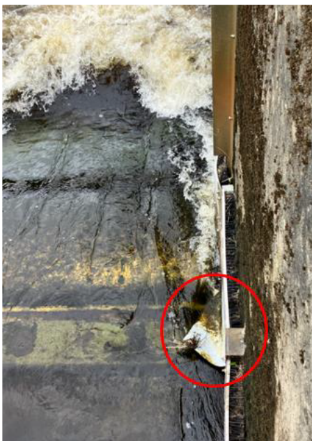
Photo 4: Damaged outer skin
