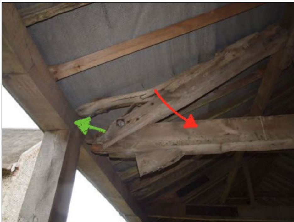
Figure 4: The roof truss has disconnected with the wall-plate and the roof has partially collapsed. Red arrow: Movement of the truss downwards. Green arrow: Movement of the wall-plate outwards (Photo: Nicholas Warns Architects).
