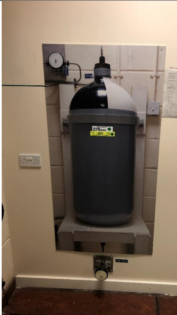
Existing “mock-up” HP air bottle – room K5C lab 2
