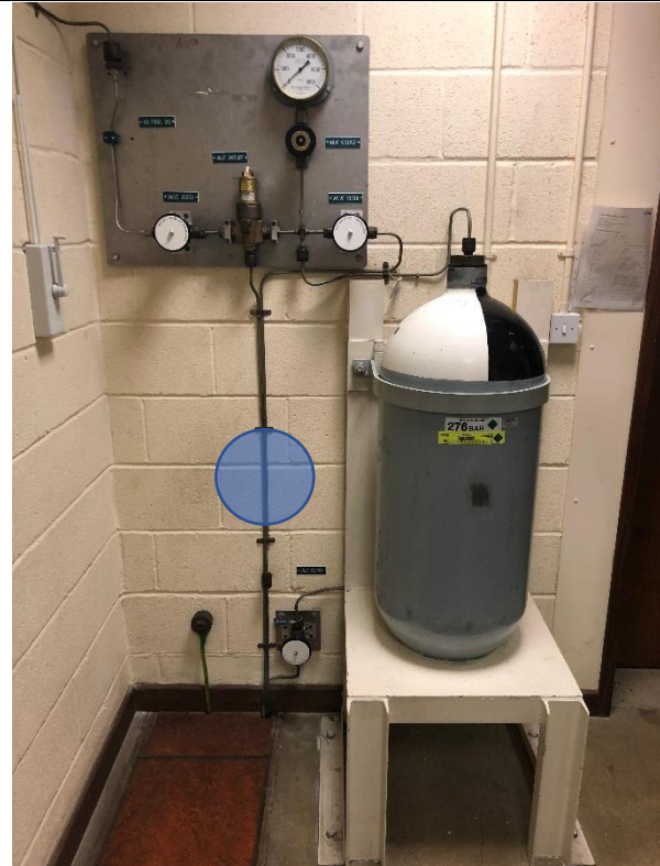
Location of double block & bleed valve isolation – room K5C lab 1
