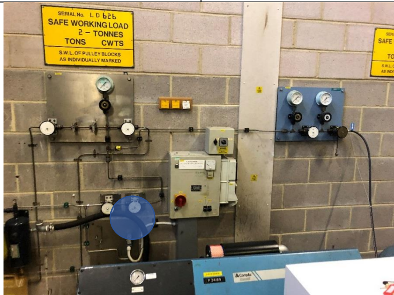
Location of double block & bleed valve isolation – room K5C lab 1
