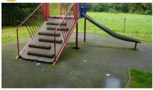
Equipment unsafe. Surface damaged with littering and moss present.
