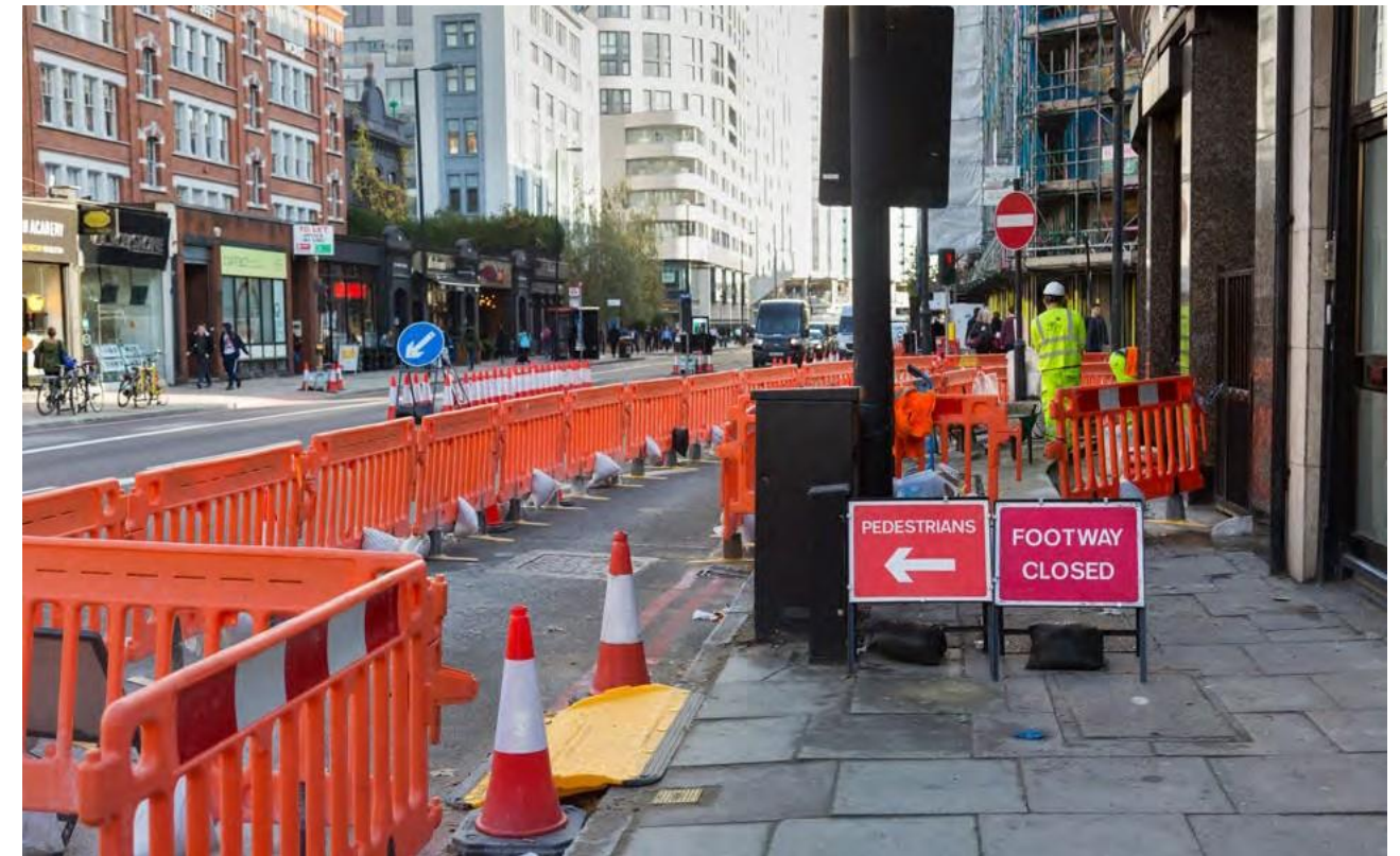
Closed footway with temporary walkway in carriageway
