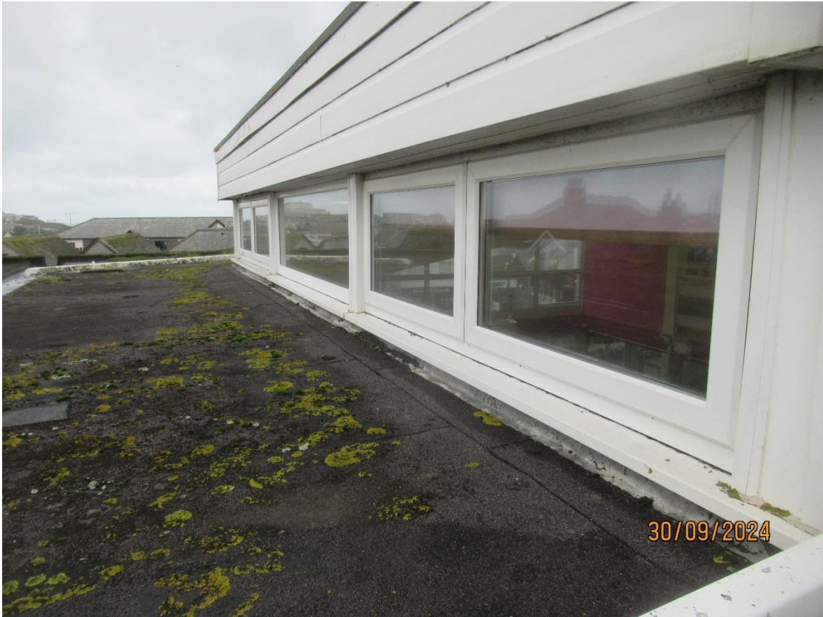
P18 – Window upstand roof three
