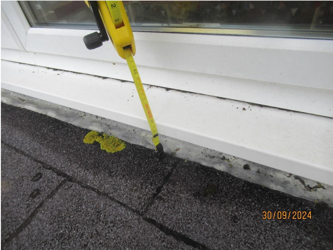
P19 – Window upstand roof three
