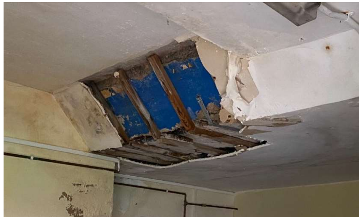
Figure 9 – Roof slab condition
