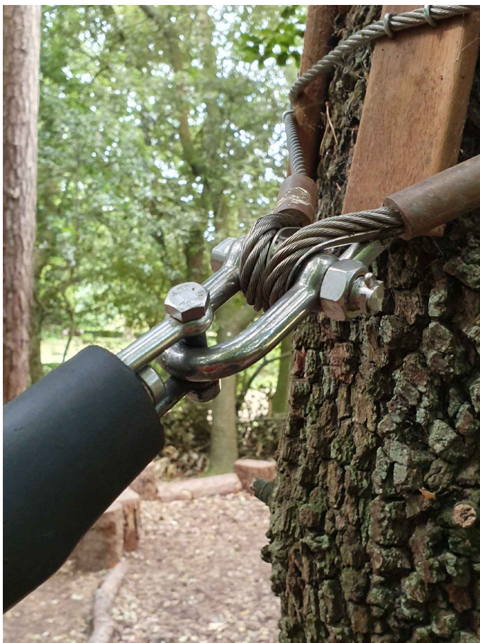
End of hammock fixing as supplied by manufacturer. Fixing shackle to connect hammock to marine grade steel rope 10mm diameter (TBC) as per manufacturers recommendations
