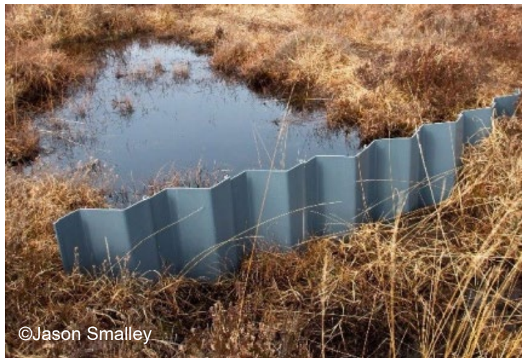
Figure 19 Plastic piling in a raised bog (Thom, 2019)
