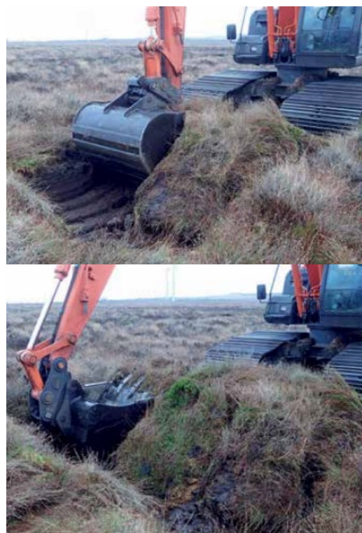
Figure 11 Creation of a wave dam (Short & Robson, 2016)
