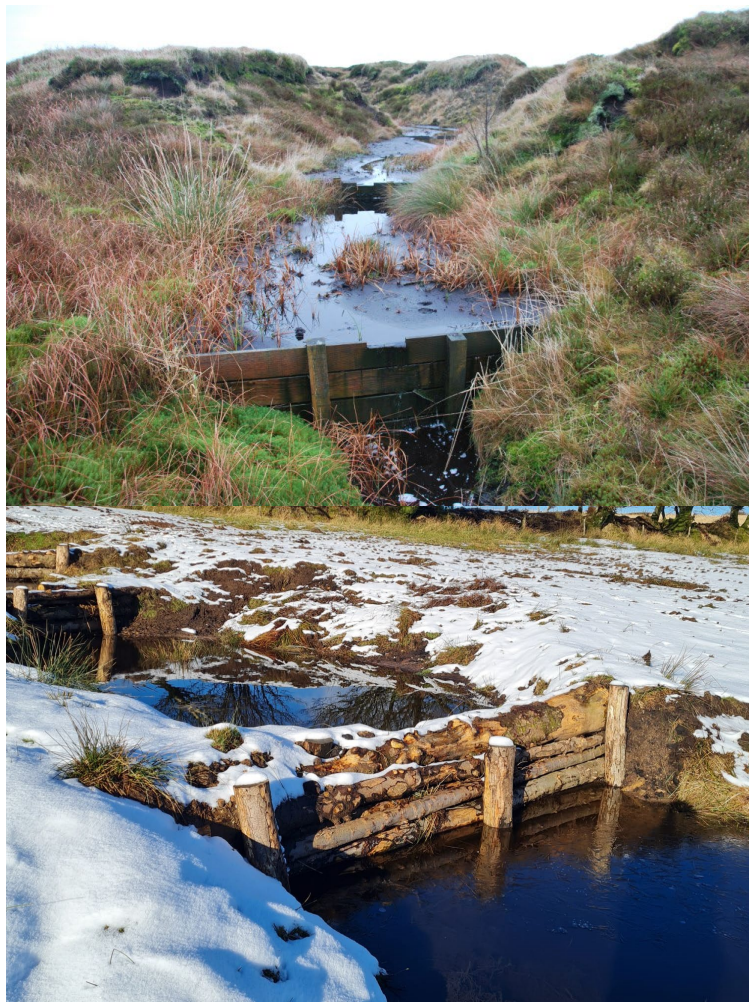
Figure 13 Top: Semi-permeable timber dams in a blanket bog gully. Bottom: Permeable dam constructed from logs. Photo credit: Moors for the Future and Deborah Land
