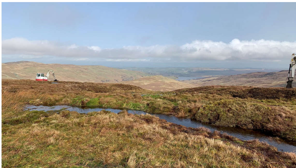
Figure 5 Top: Newly created arc bund on degraded blanket peat constructed above a large erosion gully to slow the movement of water through the peat. Photo credit: Deborah Land.
