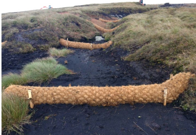
Figure 16 Coir rolls on Pendle Hill, Lancashire. Photo credit: Conservfor Ltd
