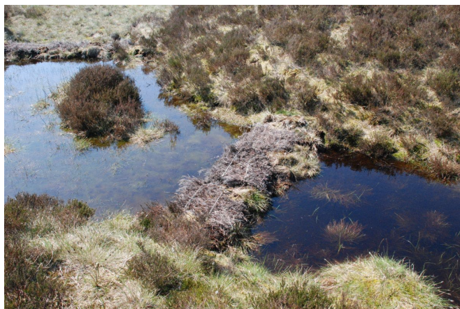
Figure 15 Established heather bale dam. Photo credit: Moors for the Future.
