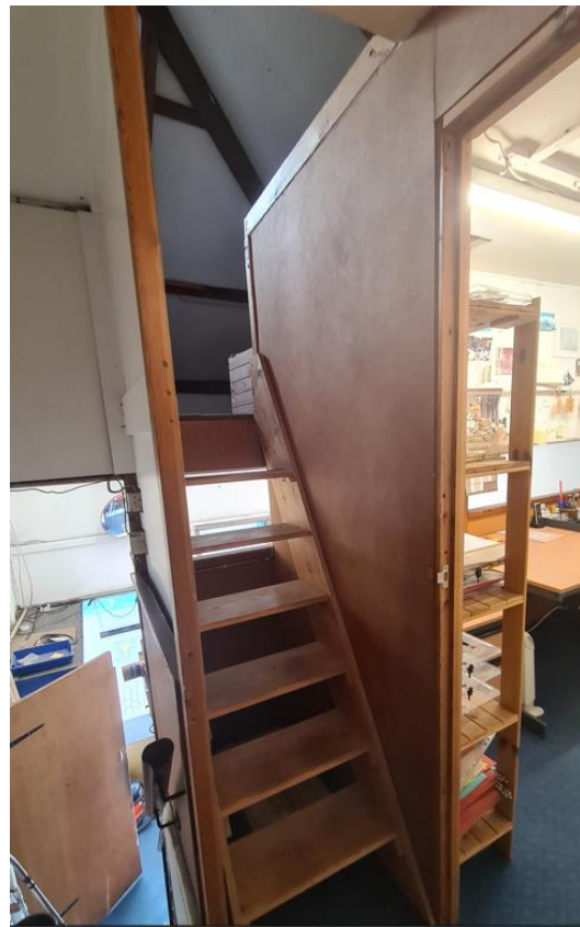
Existing stair access to attic room
