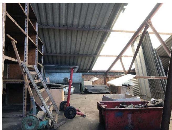
Photograph 33 - Mezzanine Floor of Unit 5 Extension with Loose Sheets of Asbestos
