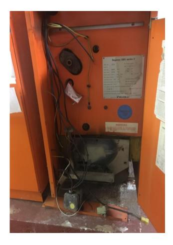
At some time in the past the gas supply for boiler No. 5 has been disconnected and utilized to supply gas an appliance not located in the main plant room.
