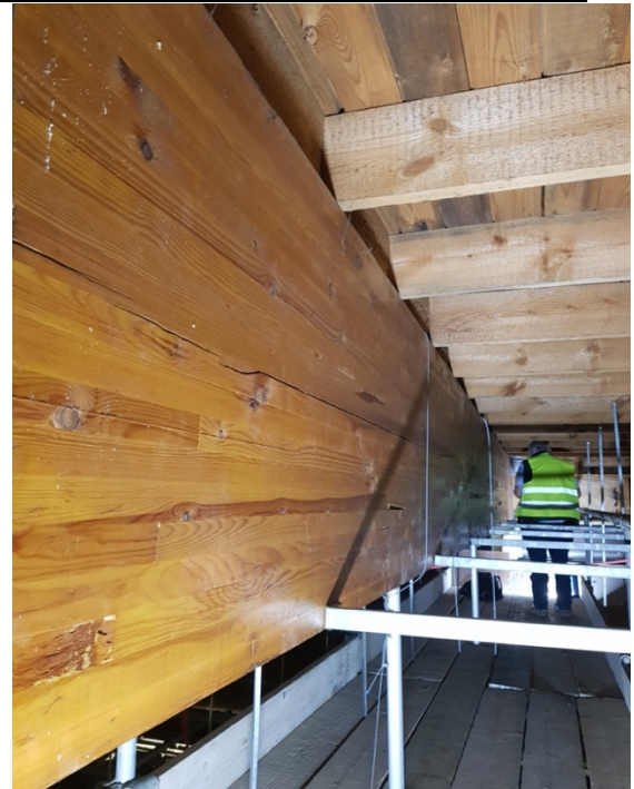
R22 Beam 3 – Horizontal check / crack
