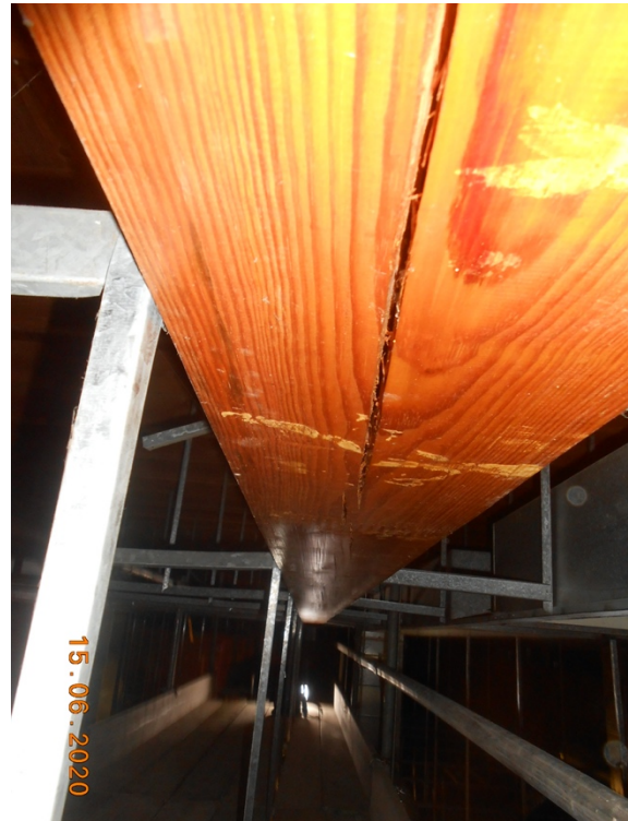
R26 Beam 3 – Fracture to beam soffit
