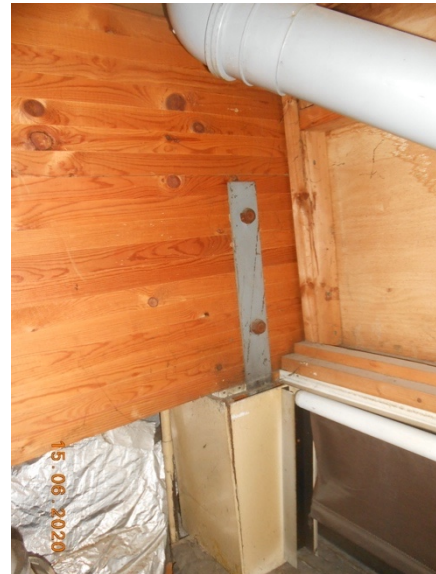
R14 Laminated beam onto ply cased post
