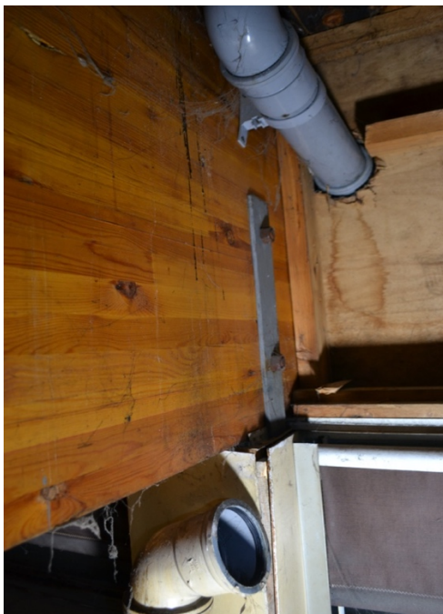
R15 Re-routed rainwater downpipe at laminated beam bearing
