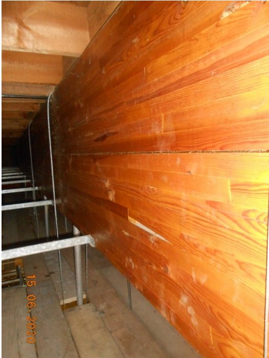
R21 Beam 3 – Horizontal crack
