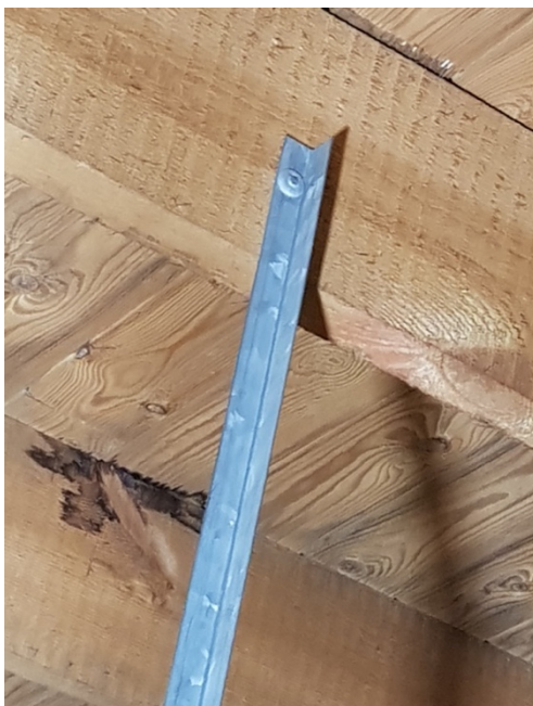
R11 Typical screw fixing for ceiling hanger
