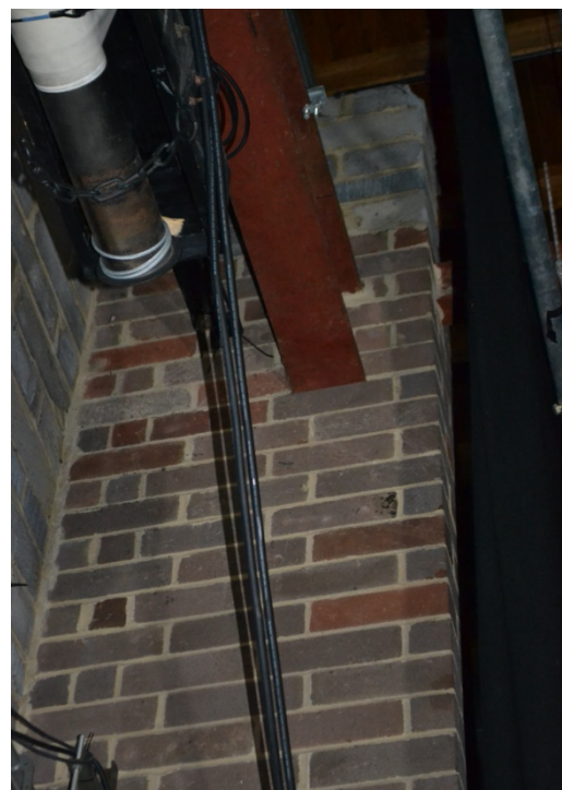
R36 Proscenium beam bearing
