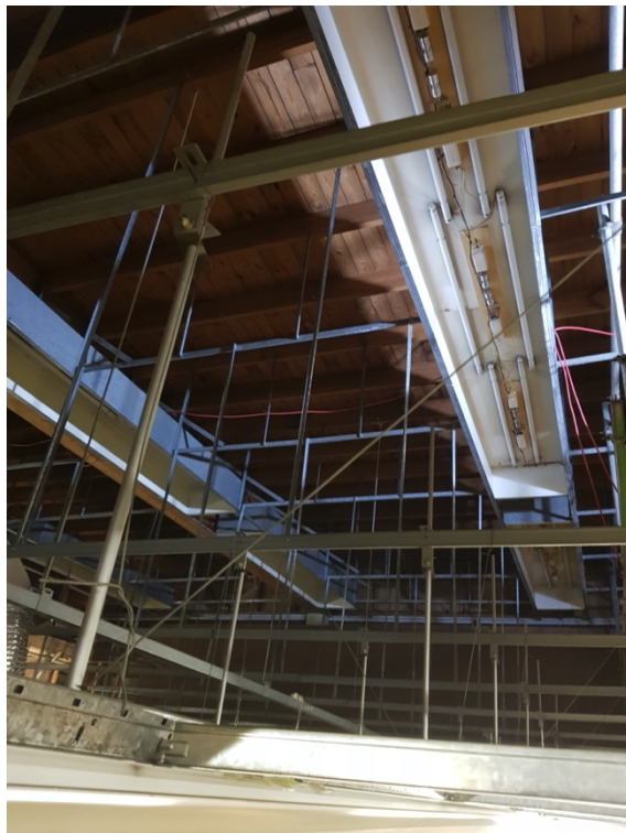
R31 Ceiling grid and redundant lights
