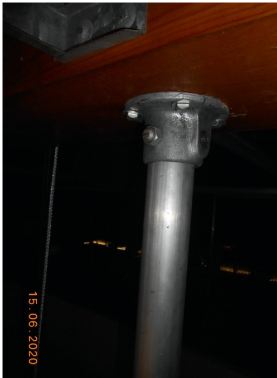
R25 Lighting bar fixing
