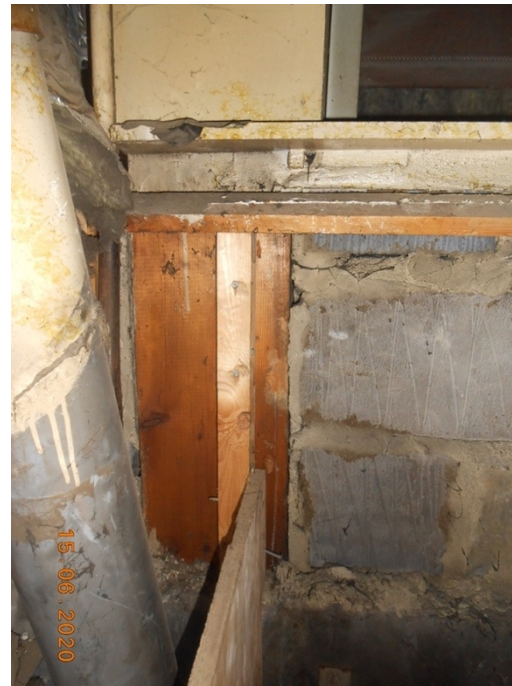
R16 Timber post below Glulam beam bearing
