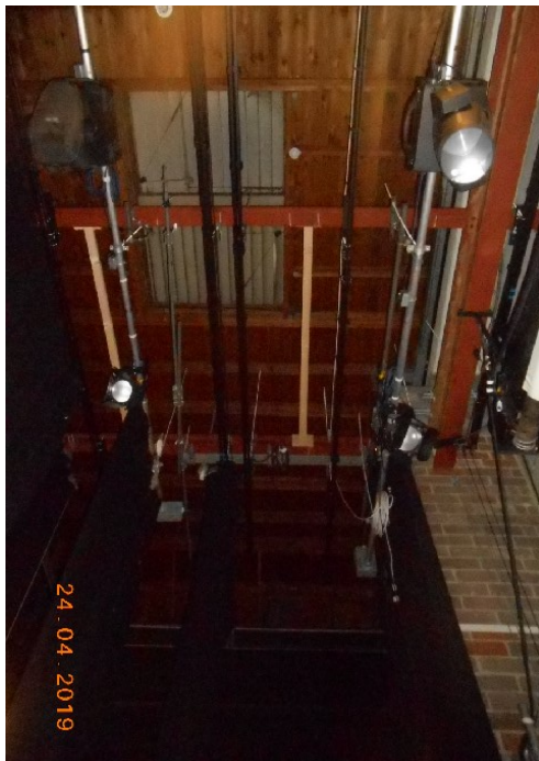
R33 Light grid. Support above stage.
