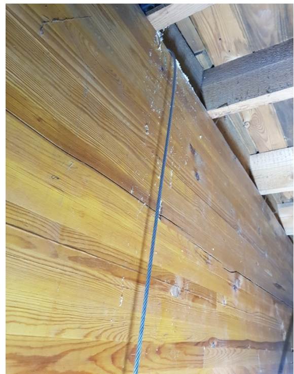
R24 Beam 3 – Safety wire
