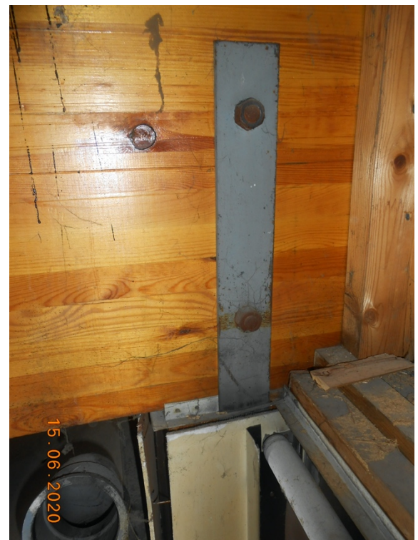
R20 Laminated beam post fixing
