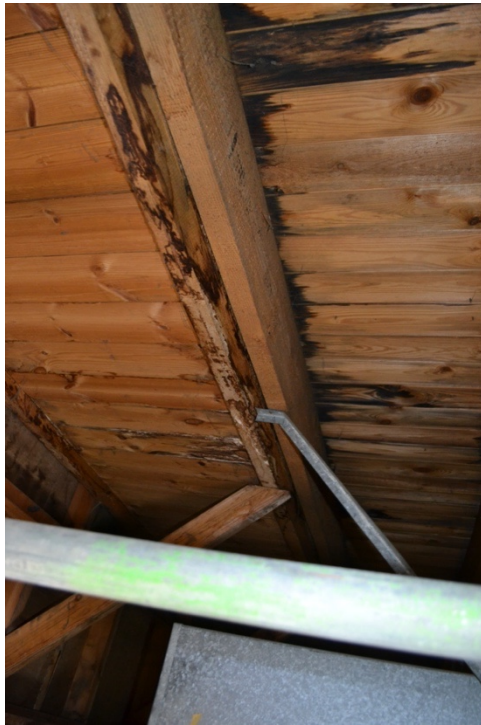
R9 Roof edge beam. Historic water penetration.
