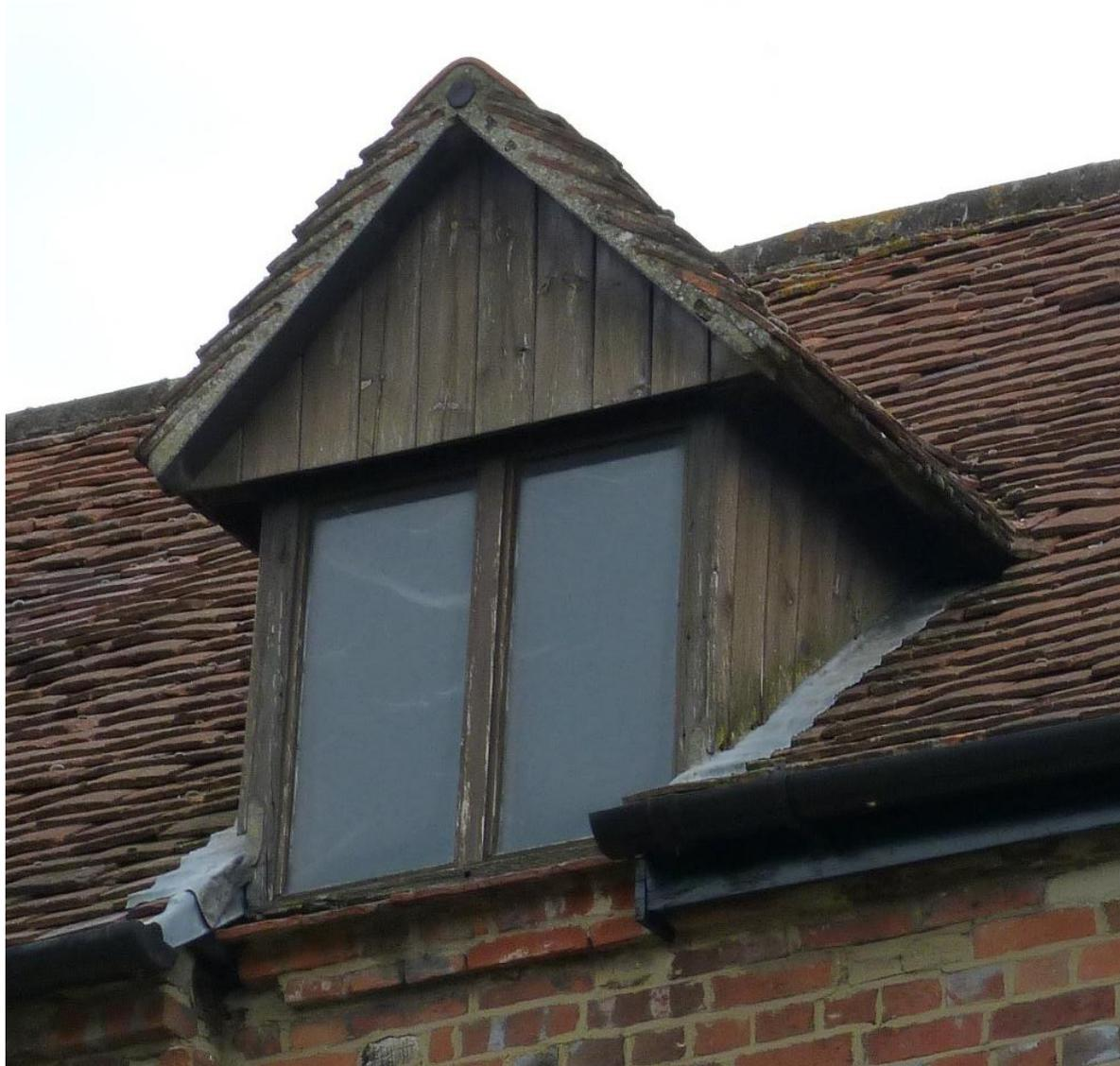
lead flashings and soakers to be inspected and replaced as necessary with code 4 lead to match existing
