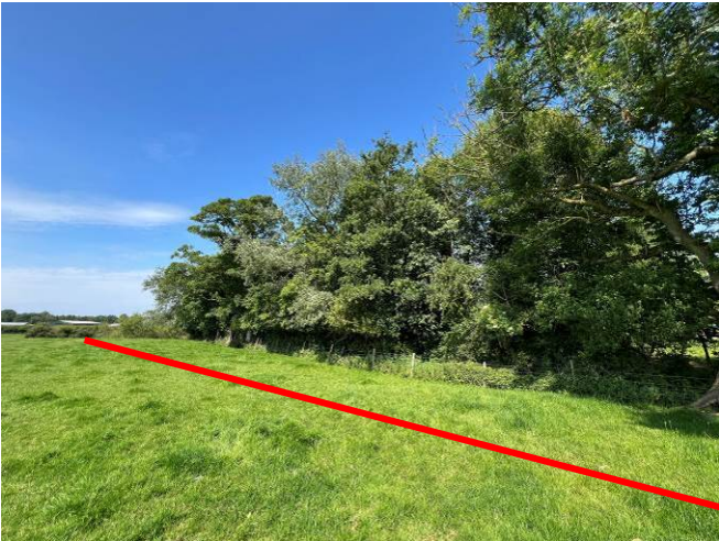
Looking west along the approximate culvert line from Browns Lane.
