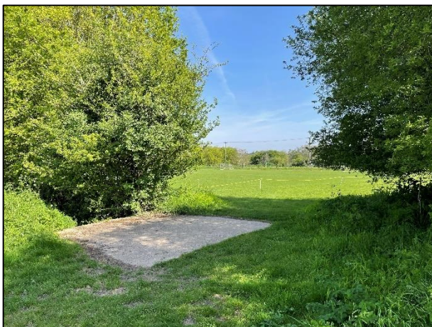
Figure 10. Concrete bridge over a ditch that runs along the south-eastern boundary.
