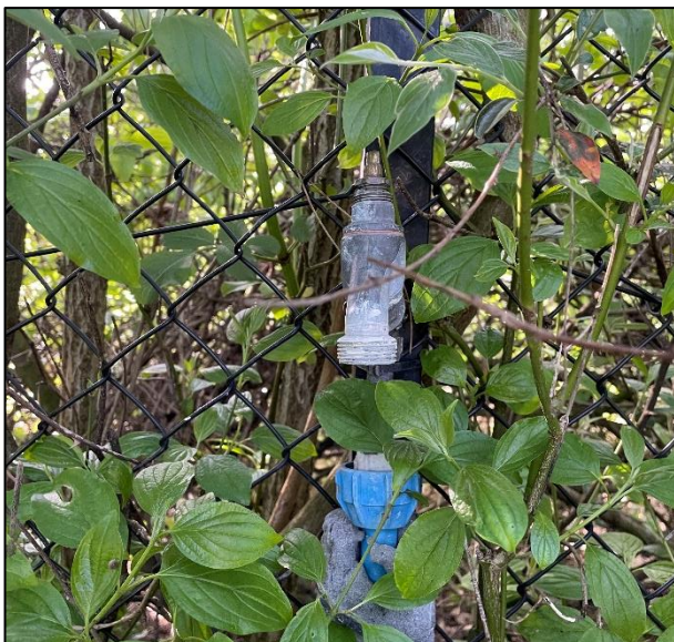
Figure 55. The north-western standpipe.
