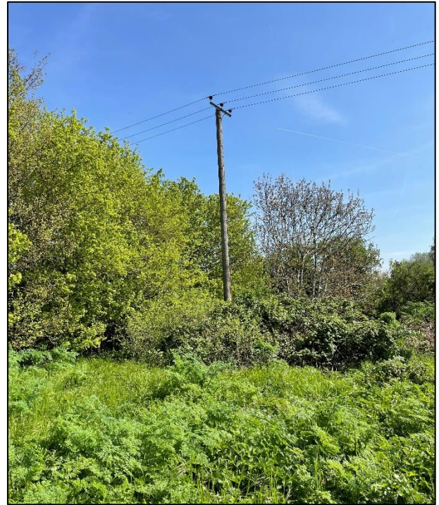
Figure 19. Overhead power lines in the fallow triangular area..
