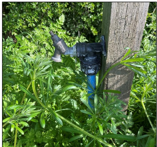
Figure 56. The southern standpipe.
