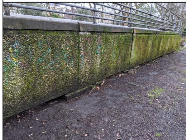
**Elevation of mass concrete pads to perimeter wall units**
