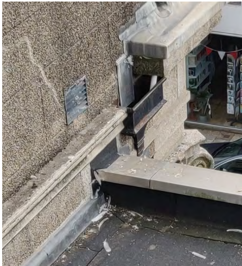
8. Poor detailing around hopper and lead.
