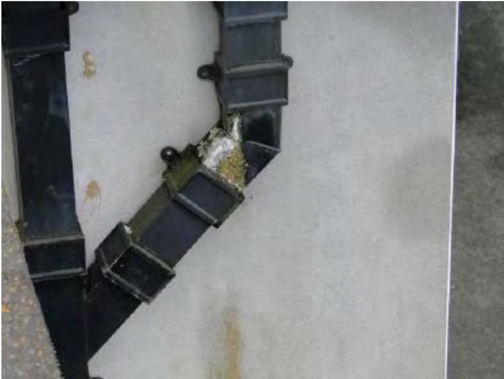
11. Typical defect to rainwater goods along north side.
