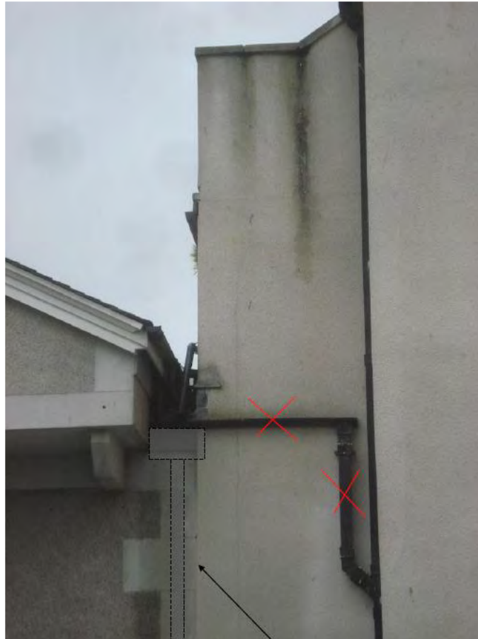
13. Location of new rainwater outlet and hopper to replace poor gutter and downpipe arrangement between R5 and R7.
