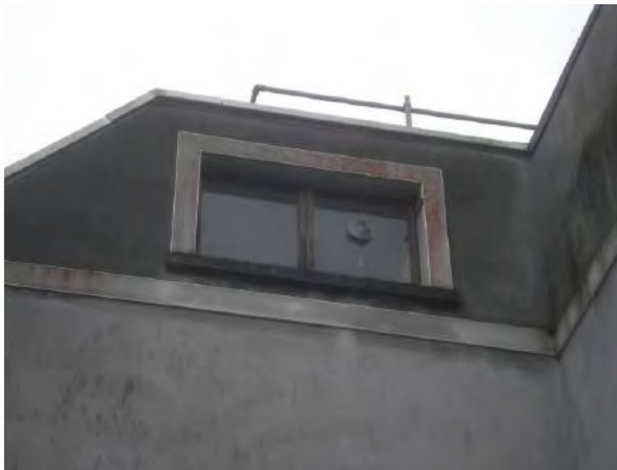
14. View of west window below S3 west side to be replaced with matching timber frame window – C20 window.
