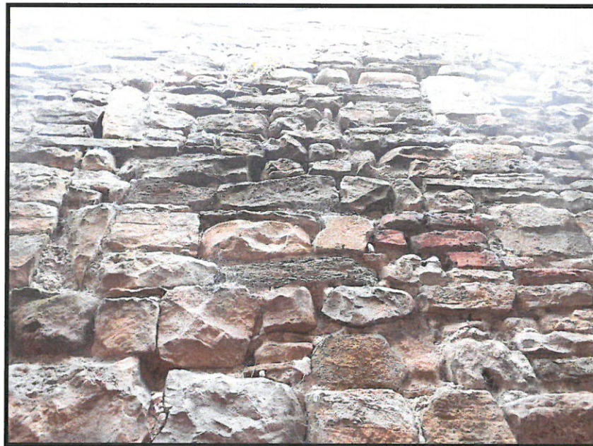
Photographs 03 & 04 Showing eroded stone & typical deterioration of mortar joints
