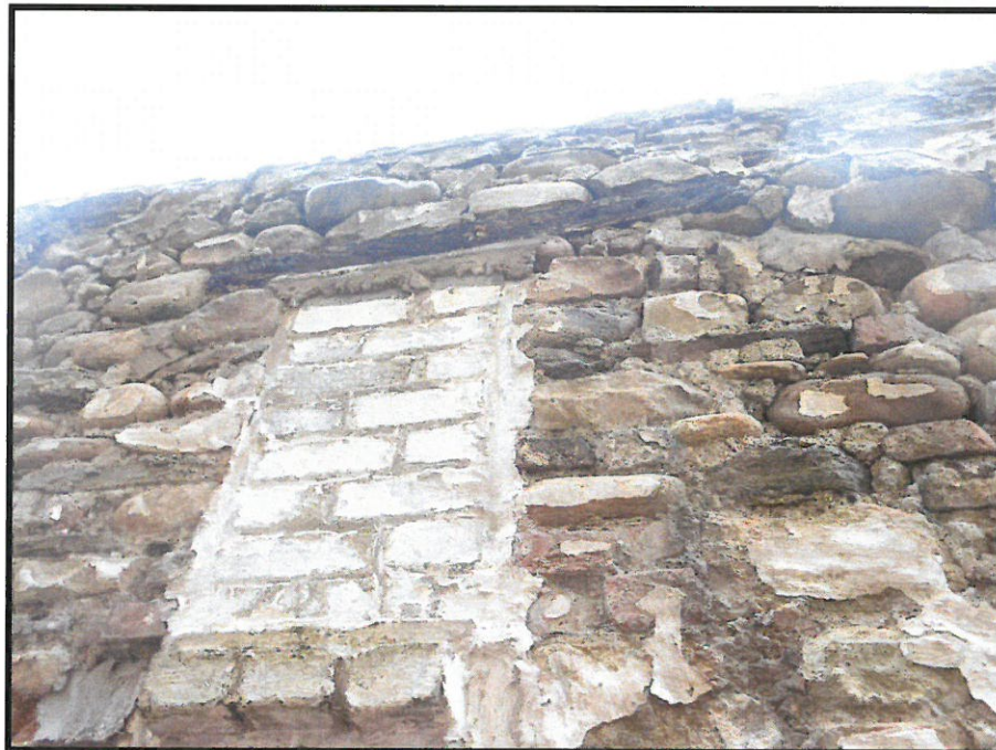
Photographs 07 & 08 Showing deterioration of embedded timbers and disruption of supported masonry
