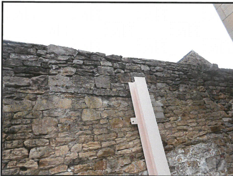
Photograph 06 Showing deterioration of mortar joints to upper wall section
