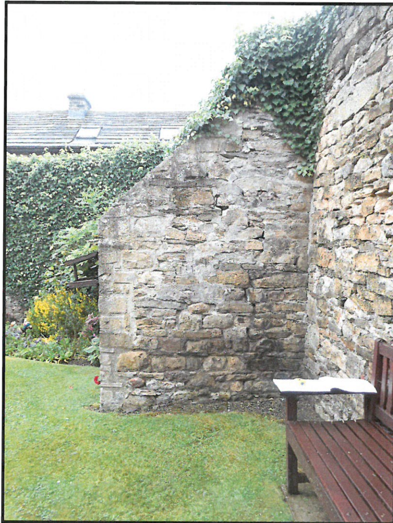
Photograph 09 Showing deterioration cracking to stone buttress
