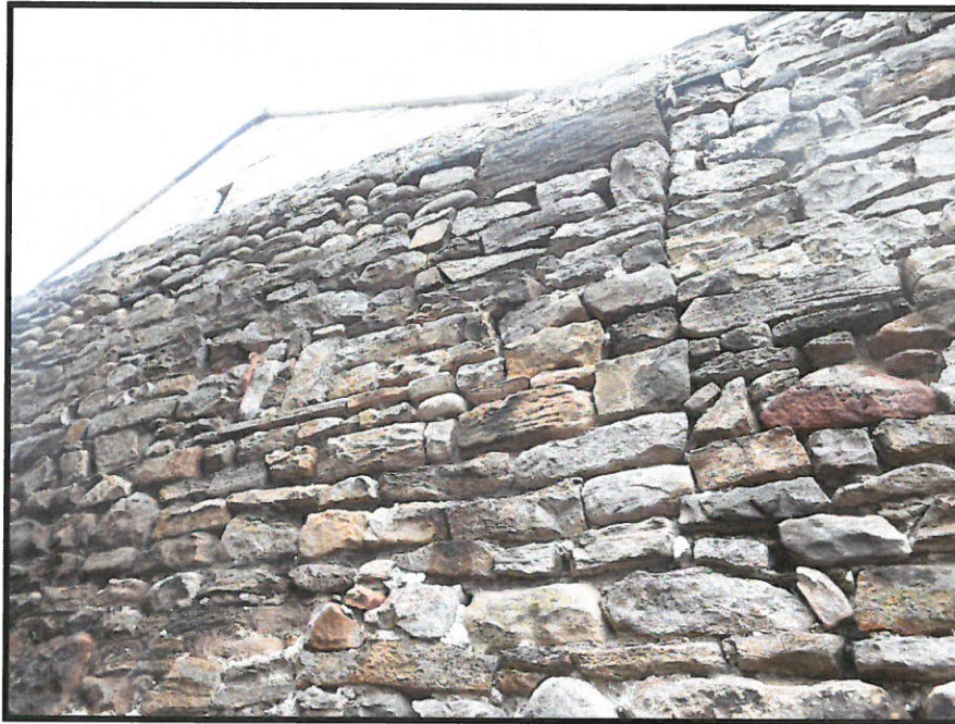
Photographs 05 Showing typical deterioration of mortar joints to infill sections
