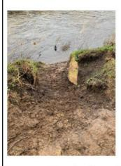
Large – Greater than 1m across in breadth - embankment rutting to be dug out to 0.5m either side of rutting, benched infill into existing slope – bench height not to exceed 500mm in height, scour protection to be provided in accordance with the Environment Agency Operational Instruction 110\_07 Technical design details for embankments, prior to covering with top-soil and reseeded with a grass seed mix that will provide an adequate grass squad and root penetration.
