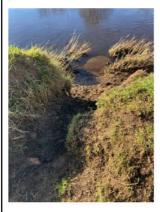
Scour protection should be provided and derived in accordance with the Environment Agency Operational Instruction 110\_07 Technical design details for embankments. The ground should be restored to the level of the existing embankment.
