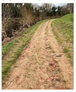
Asset 763796 Repair and reinstate Track Section 5 on earth embankment including edging board replacement.
