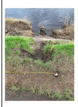
Medium – Around 1m across in breadth - embankment rutting to be dug out to 0.5m either side of rutting, benched infill into existing slope – bench height not to exceed 500mm in height, scour protection to be provided in accordance with the Environment Agency Operational Instruction 110\_07 Technical design details for embankments, prior to covering with top-soil and reseeded with a grass seed mix that will provide an adequate grass squad and root penetration.
