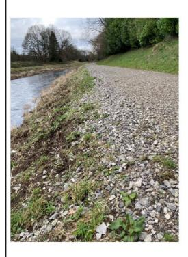
Asset 121968 Repair and reinstate Track Section 6 on earth embankment including edging board replacement.
