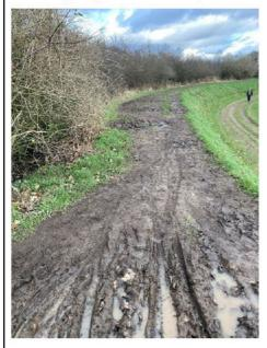
Asset 763795 Earth embankment section of meander erosion.
