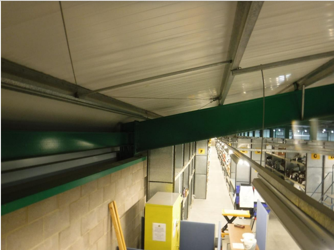
Digital Image 05 – General View of Rafter and Purlins
