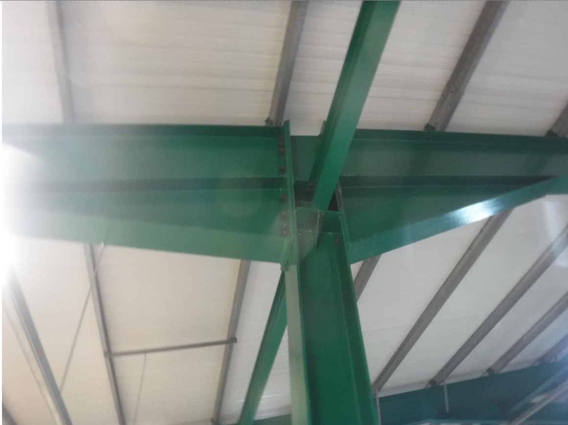
Digital Image 04 – General View of Column & Rafter Connection
