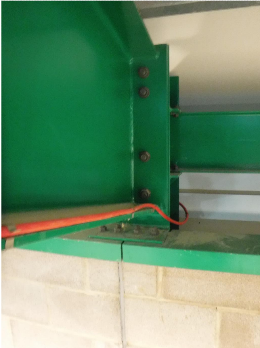
Digital Image 06 – General View of Eaves Detail
