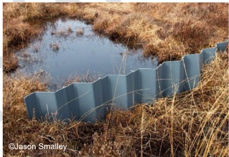
Figure 19 Plastic piling in a raised bog (Thom, 2019)
