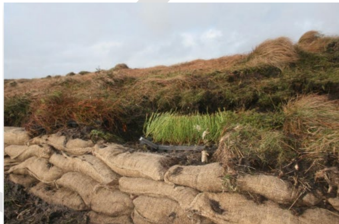
Figure 20 Soil-filled jute bags laid stretcher bond about to be plug planted, Blackstone Edge Roman Road. Photo credit: Moors for the Future 2015
