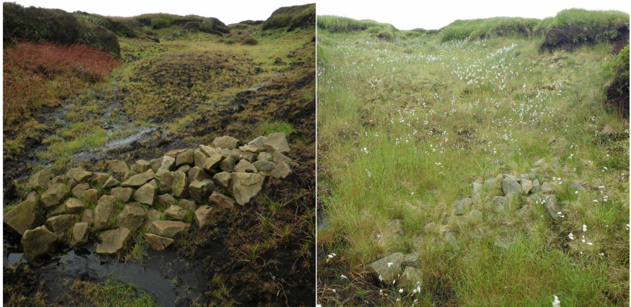
Figure 14 Stone dam installed in the Peak District. Photo Credit: Moors for the Future
