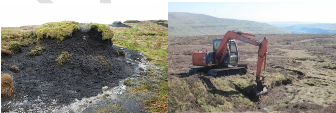
Figure 21 Top: Peat hagg. Bottom: Reprofiling of a hagg. Photo credit: Cumbria Wildlife Trust
