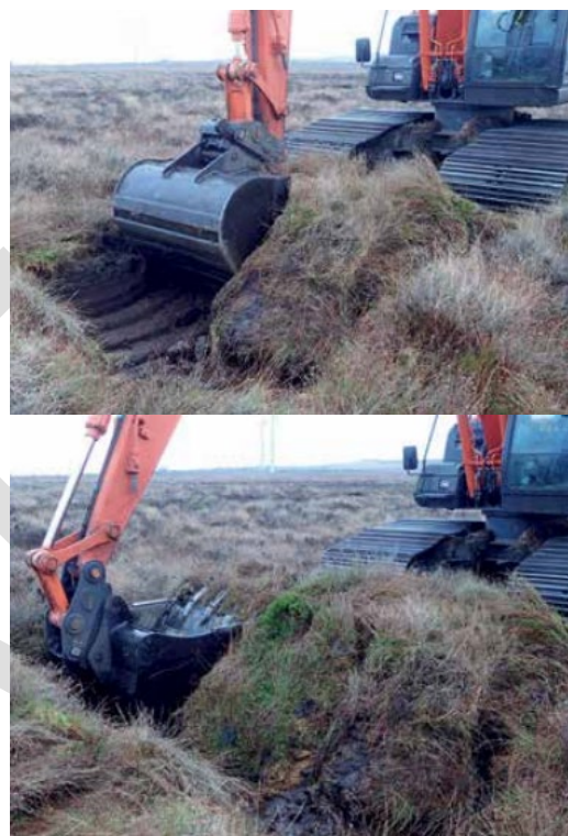
Figure 11 Creation of a wave dam (Short & Robson, 2016)
