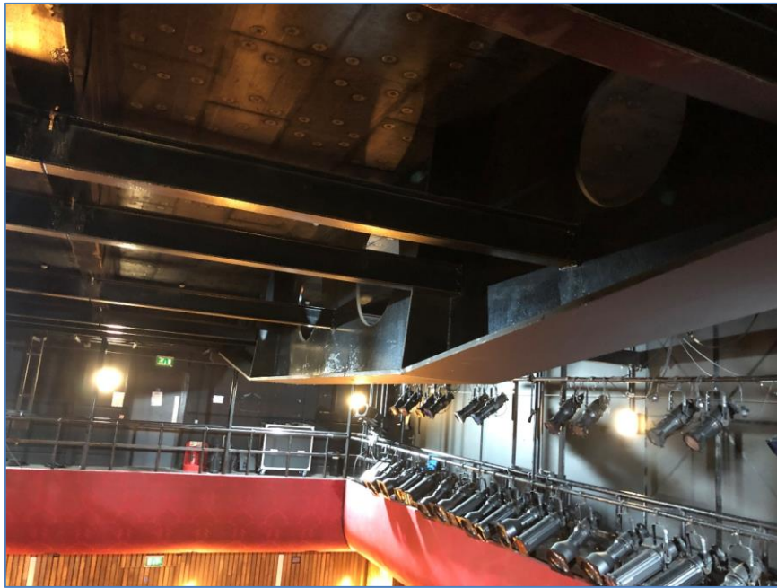
Figure D1 – L01 Theatre soffit supported by steels
