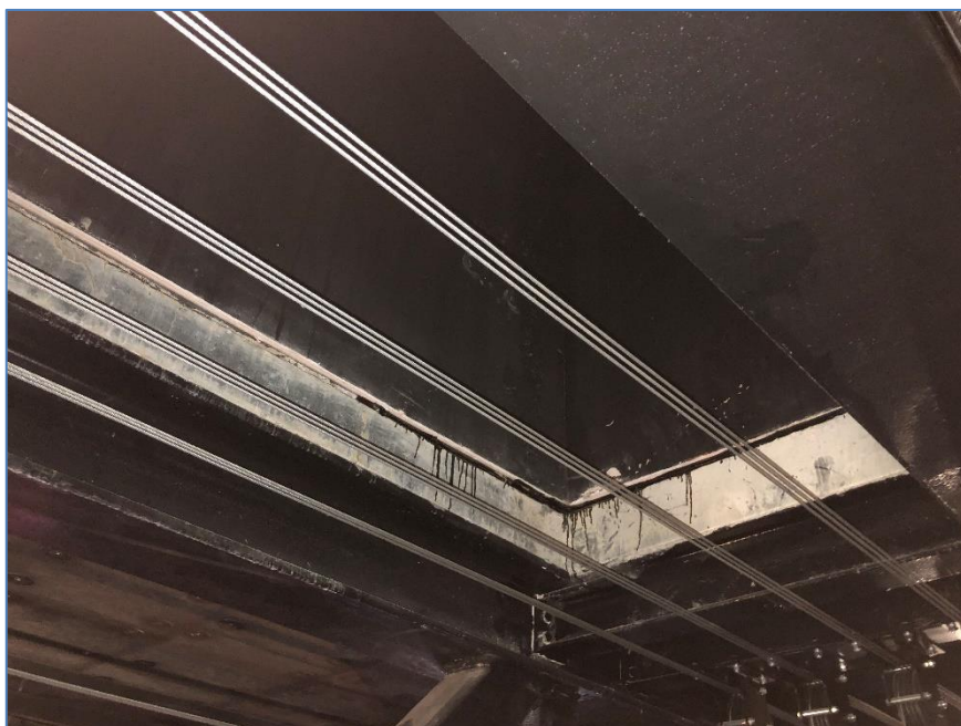
Figure D4 –Smoke extract void opening as viewed from L01 Theatre gantries above the stage
