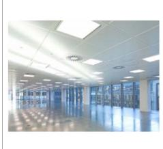
Adjusted Driver mA output to be 4000lm output.
