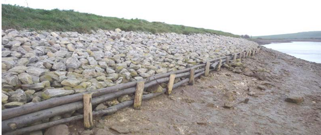
Figure 1: Completed pole-wharfing repair to tidal River Ouse embankment using Kentish Ragstone.
