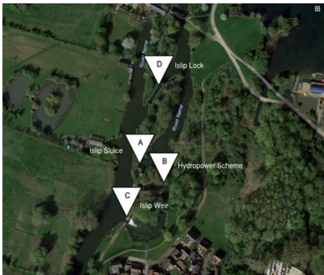
Figure 1 – Configuration of assets around Islip Sluice
