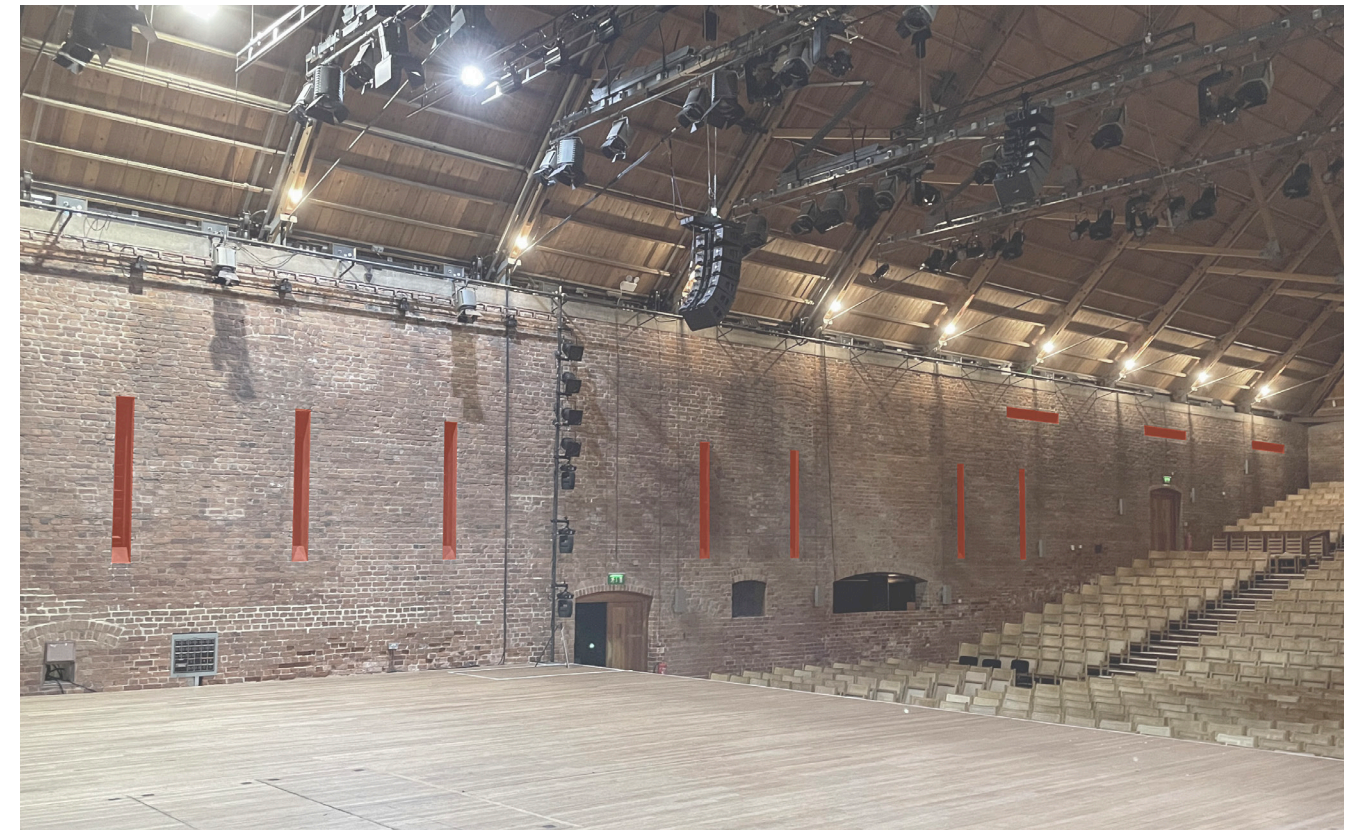
Slots within south wall of Concert Hall, through which air is blown into the Concert Hall
