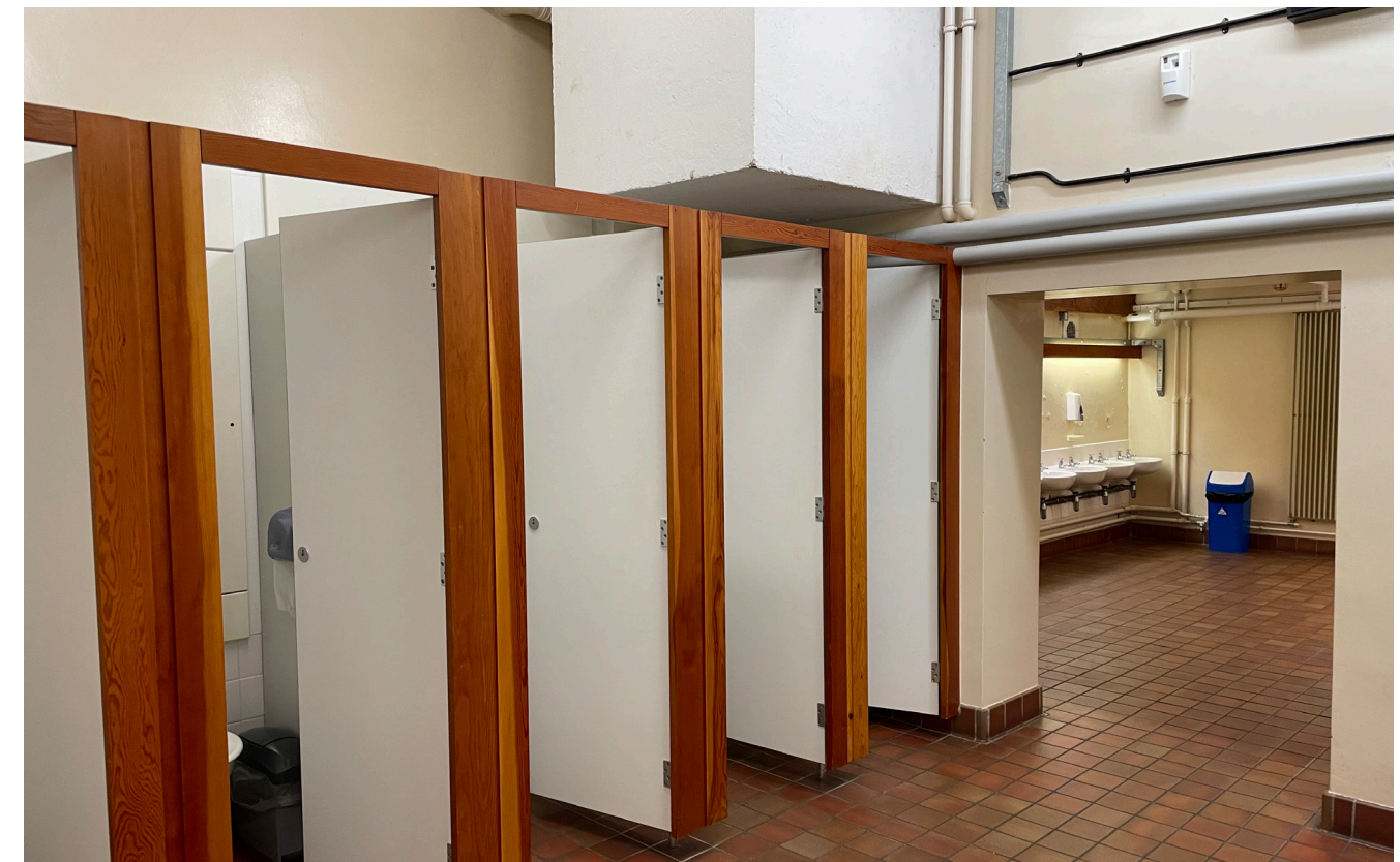
Photograph showing typical WCs as at present
