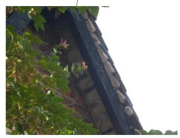
The gable end roof overhang is to be under-boarded using 18mm T & G boards painted black and an under-cloak board is to be provided under the overhanging edge tiles to allow pointing to the tile edge
