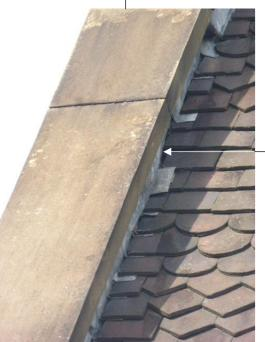
Existing stone coping blocks are to be removed to allow lead flashings to be replaced. The copings are to be replaced using stainless steel restraint angles in the joints as per SE detail
