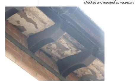
The eaves overhang soffit is to be removed and the soffit is to be boarded with 18mm T & G boards, painted black
