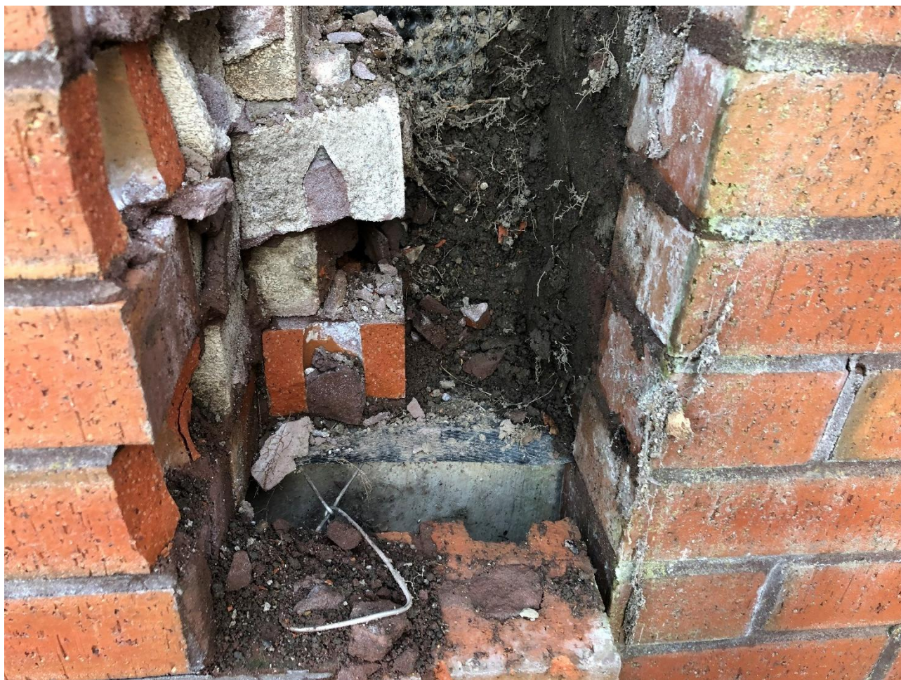
Photo 9 – Close up of exposed concrete stem
