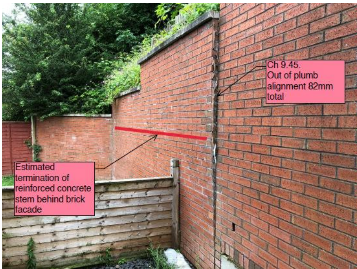
Photo 2 – Section wall showing movement
