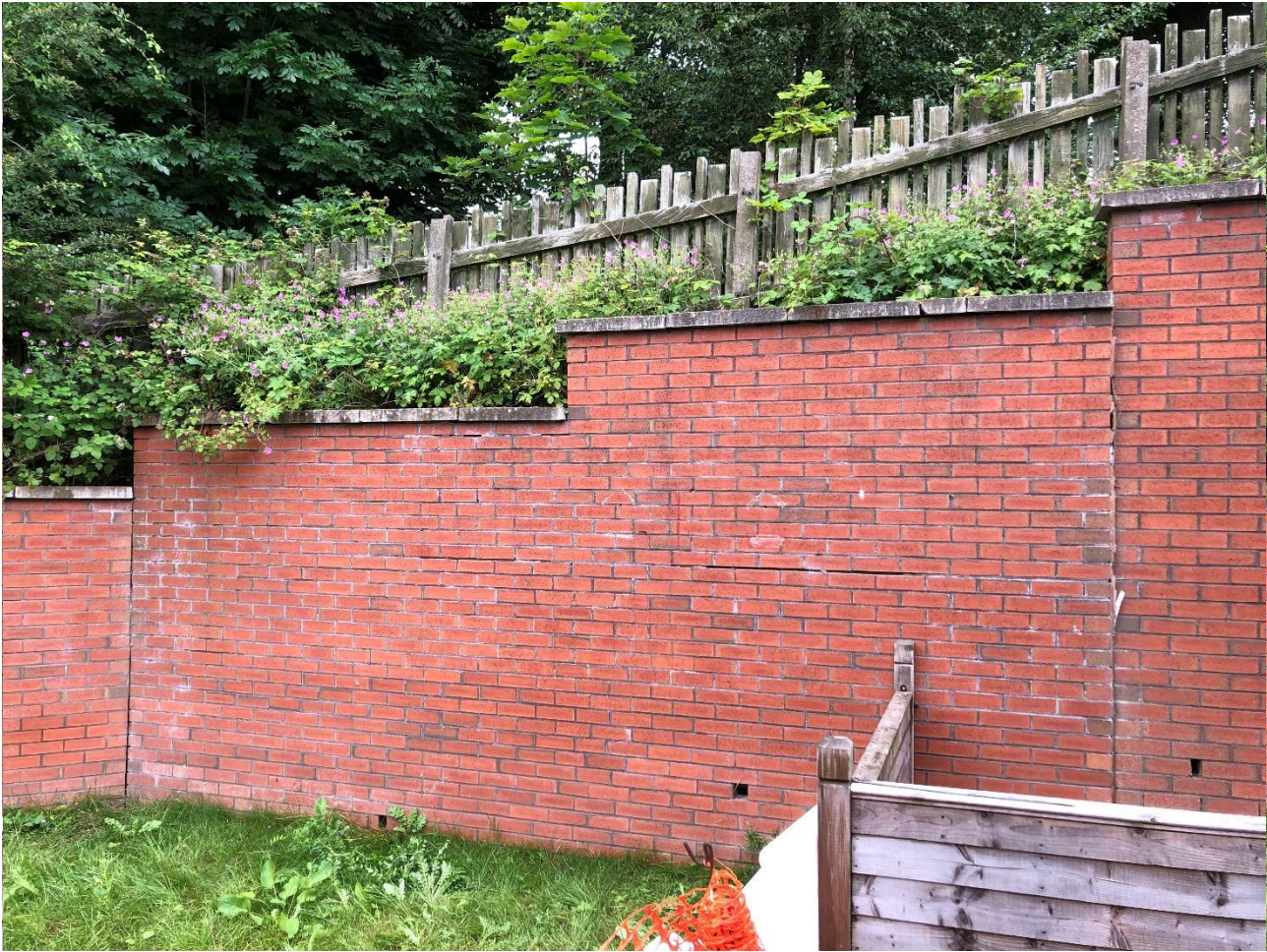
Photo 4 – Elevation of section under movement
