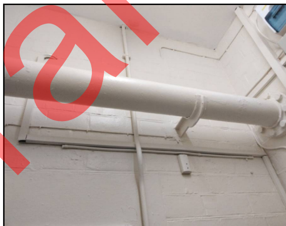
1st Floor Cleaners cupboard (36) Thermal Insulation Lagging Pipework 197
