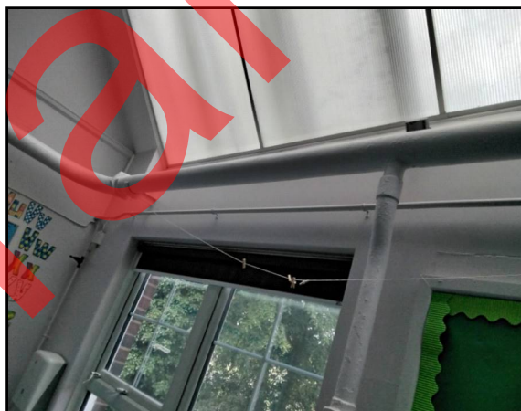
1st Floor Classroom 3B (20) Thermal Insulation Lagging Pipework 166
