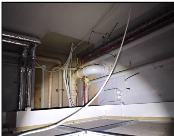
1st Floor Boys toilets (45a) Thermal Insulation Lagging Pipework 204
