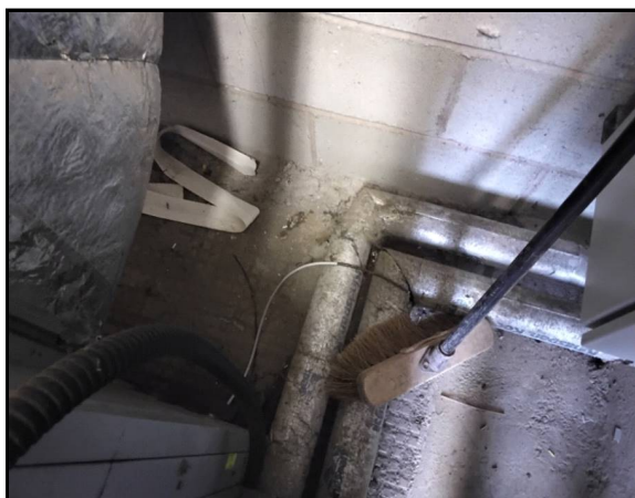
Z-Sub Level 1 Boiler room 1 (83) Thermal Insulation Lagging Floor 223
