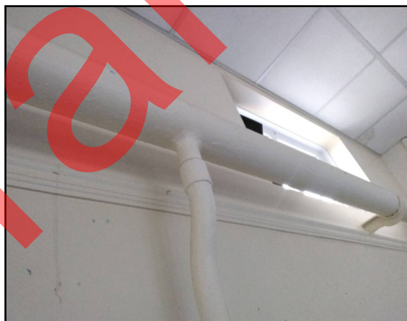
1st Floor Classroom 2C (11) Thermal Insulation Lagging Pipework 141
