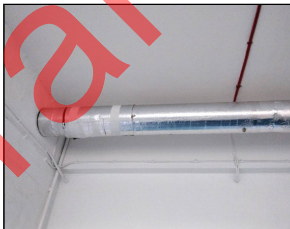
1st Floor Stairs (1) Thermal Insulation Lagging Pipework 155
