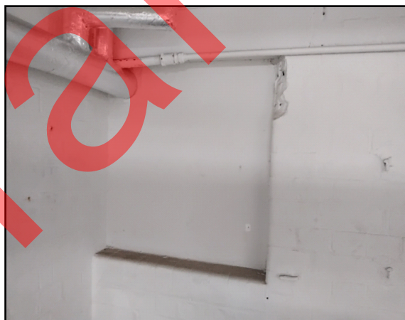
Z-Sub Level 1 Pump room (B1) Insulating Board Wall - Panel 244
