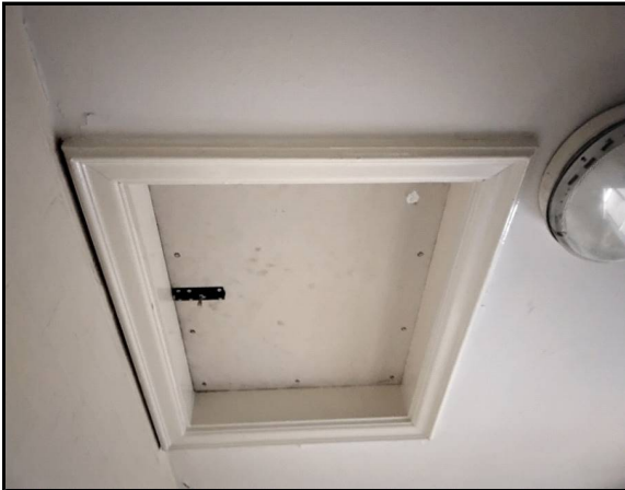
1st Floor Disable toilet lobby (81) Insulating Board Access hatch 132
