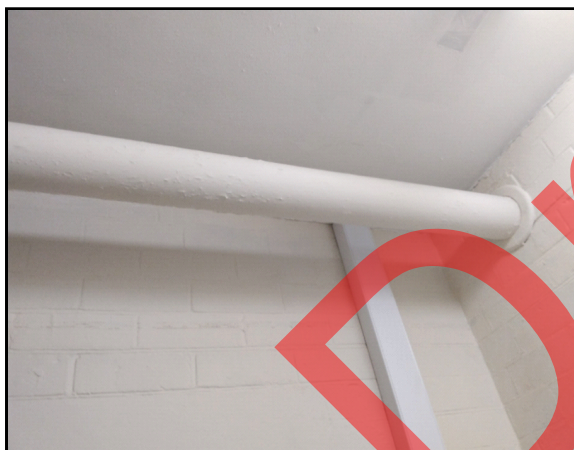
1st Floor Sensory room (2) Thermal Insulation Lagging Pipework 154
