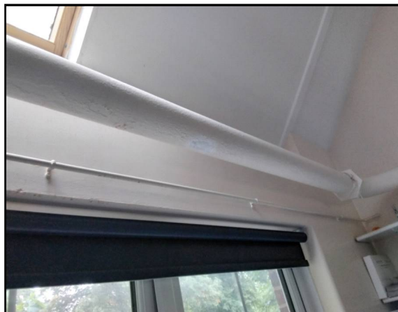
1st Floor Classroom 4S (51) Thermal Insulation Lagging Pipework 103
