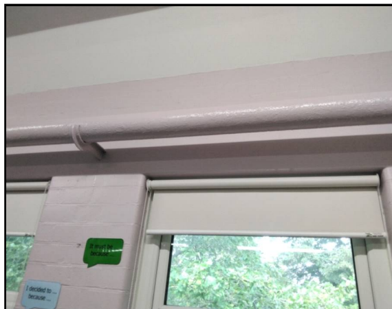
1st Floor Classroom 6B (65) Thermal Insulation Lagging Pipework 122
