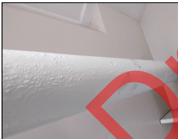
1st Floor Classroom 4ks (52) Thermal Insulation Lagging Pipework 104
