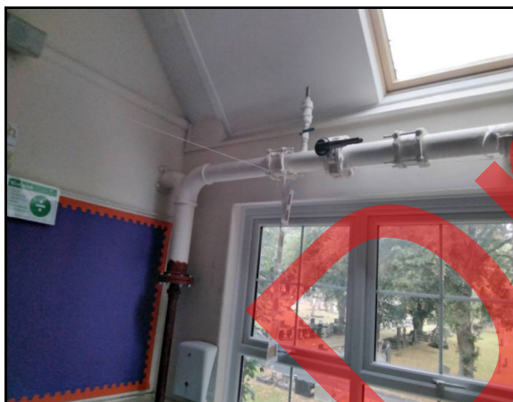
1st Floor Classroom 6T (61) Joint/Gasket Pipework Gasket(s) 117
