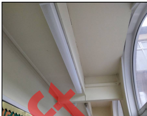
Ground Floor Corridor (32) Insulating Board Ceiling and boxing 29
