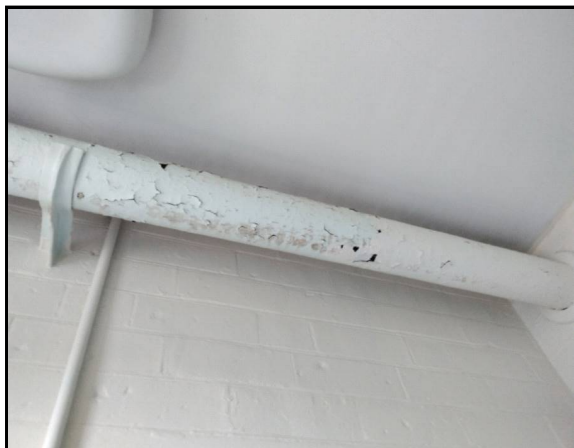
1st Floor Toilet (16) Thermal Insulation Lagging Pipework 160
