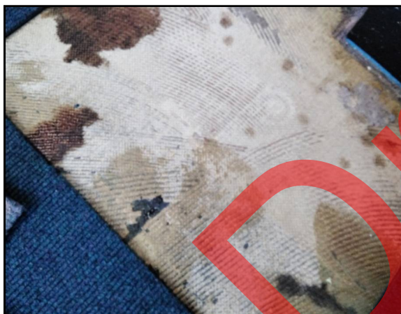
1st Floor Corridor (17.2) Composite Resinous/Reinforced Plastics Floor 182
