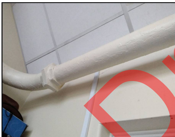
1st Floor Classroom 2B (19) Thermal Insulation Lagging Pipework 164
