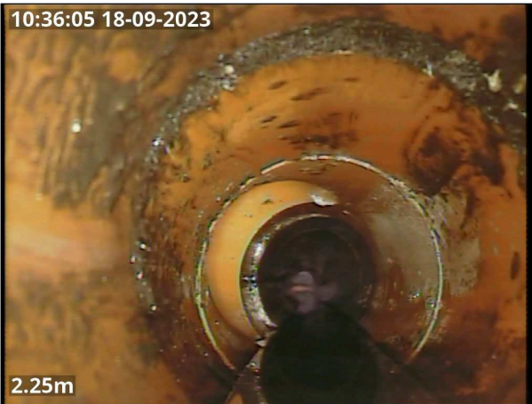
Photo: CCTV 12 pic 1.jpg 2.25m, General remark
