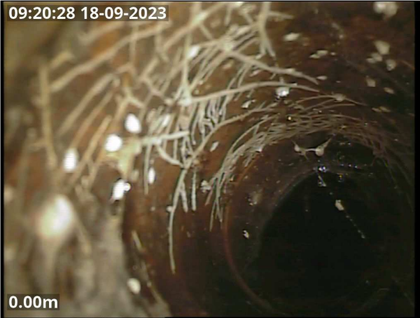
Photo: CCTV 03 pic 1.jpg 0m, General remark
