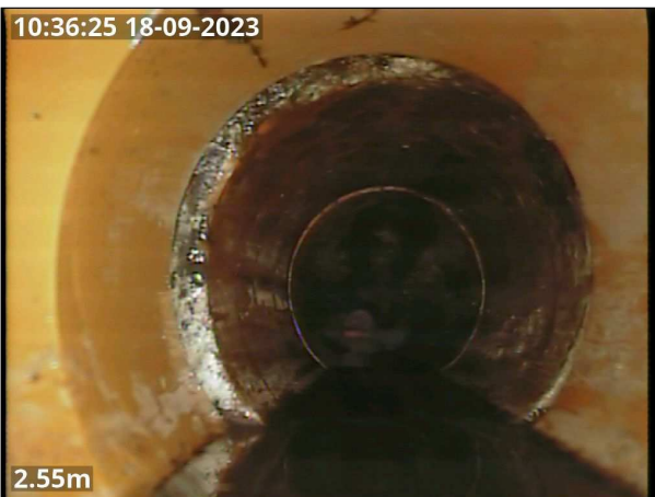
Photo: CCTV 12 pic 3.jpg 2.55m, General remark
