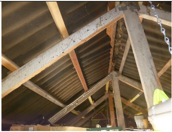
Timber framed roof structure and no sarking felt to underside of roof covering.
