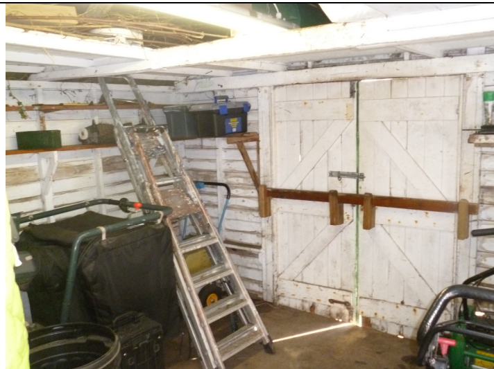
Timber inner wall structure, no wall voids and a solid concrete floor slab.
