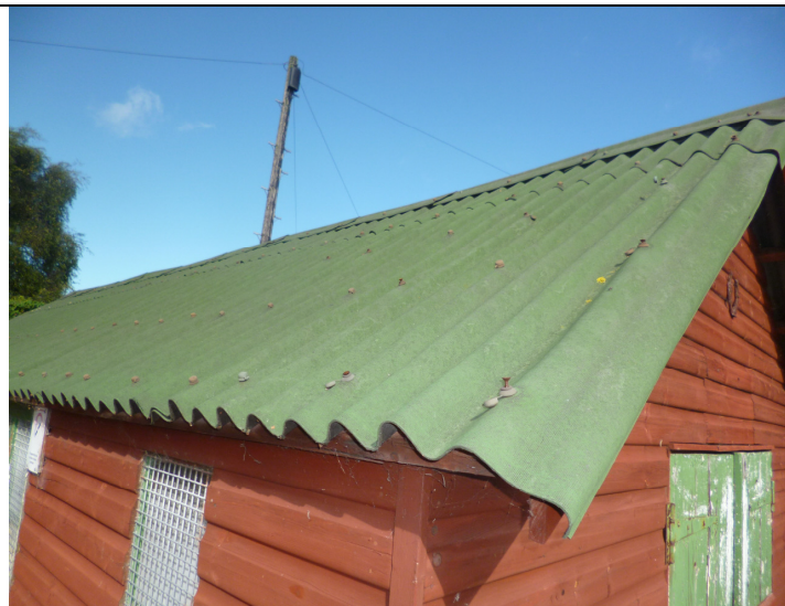
Modern fibre corrugated sheet roofing panels.
