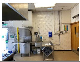
Gas pipe drop and gas stop valve where the partition is to come of the wall adjacent to the door is to be moved onto the new partition immediately adjacent
