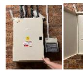
Form a plasterboard partition around this distribution board to underside of new slab above, width and depth of the plasterboard are to be sized to suit the distribution board.
