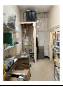
It is suggested that a timber post is incorporated in the new partition to allow a horizontal timber to span between the external wall over DG-05 and this partition post to retain the water tank platform
