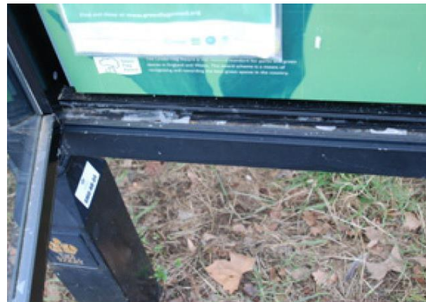
Damaged seal
