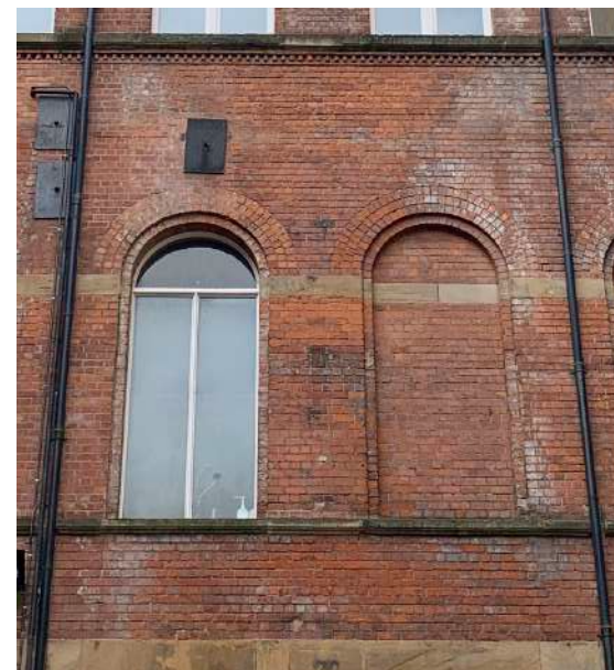
Red Brick with Stone Banding, Sills and lintels- Rear Elevation
