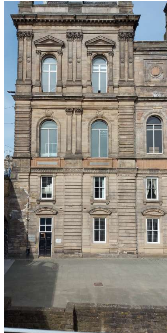
Image 1.2 - Canada House South East Elevation, Shude Hill
