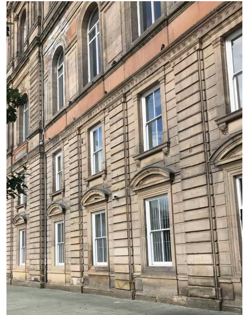
Image 1.3 - Canada House South East Elevation, Shude Hill
