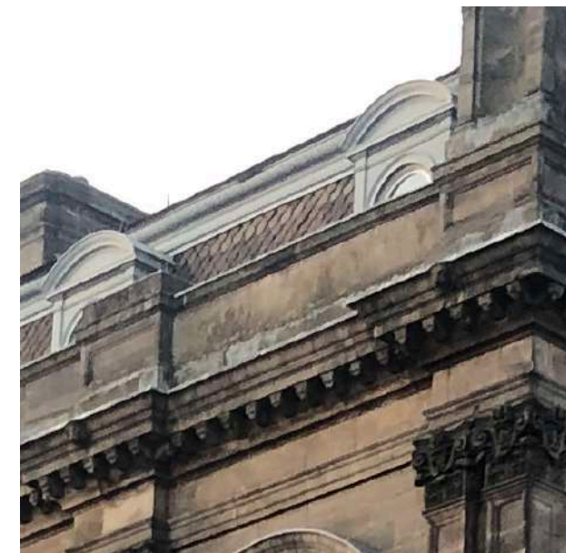
Slate Tile Shingles - Lower roof Area
