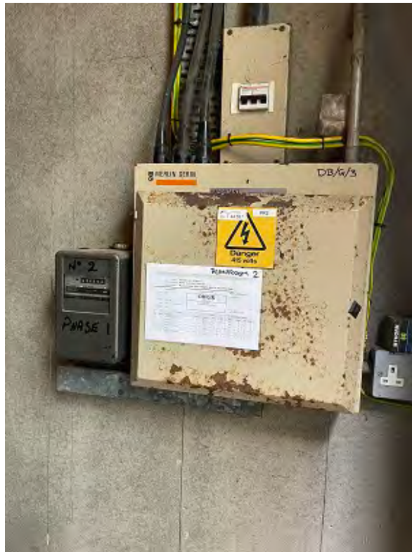
3 Corrosion damage to external plant room
