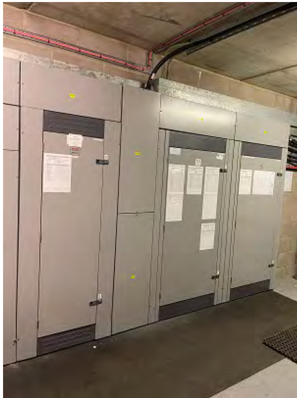
11 Cobham Hall main electrical switch panels
