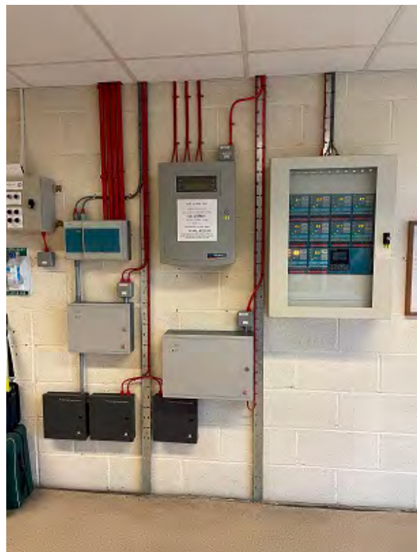
10 Cobham Hall fire alarm panels
