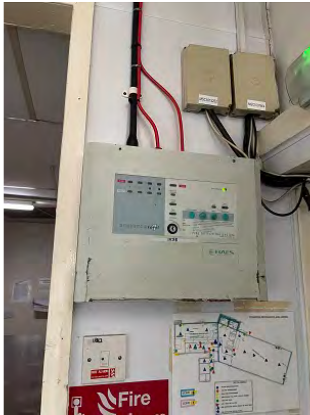
7 Swordfish Building fire alarm panel with impact damage to casing
