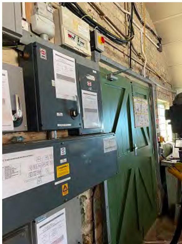
8 FM Workshop main electrical switchgear
