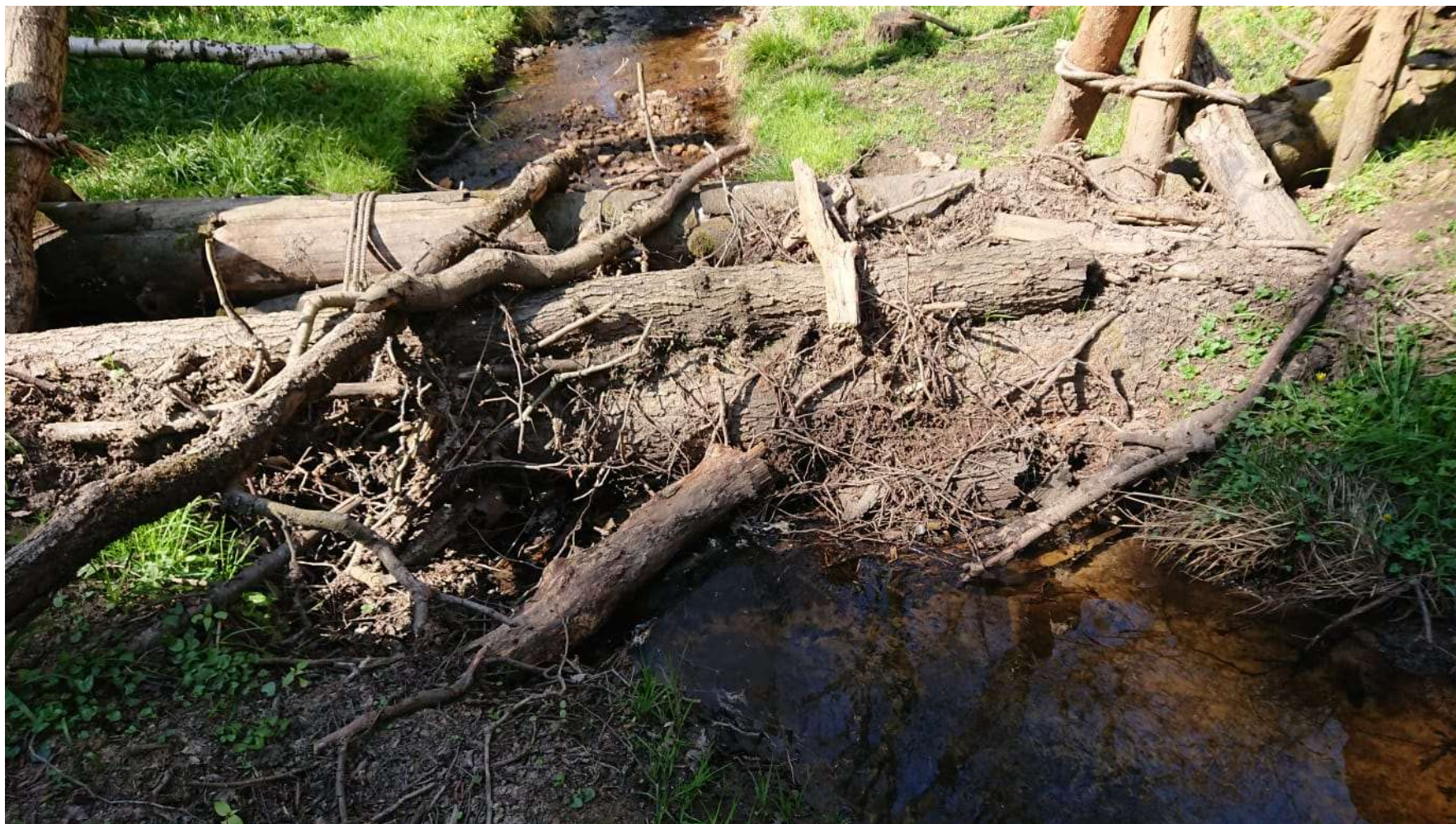
Photo 17 1b.1; 2b; 3b.1 Represents an example of what has been constructed at other sites using NFM principles. As stressed in the specification, it will depend on the character of the watercourse, what we want the dam to achieve, and the contractor's creativity and capability.
