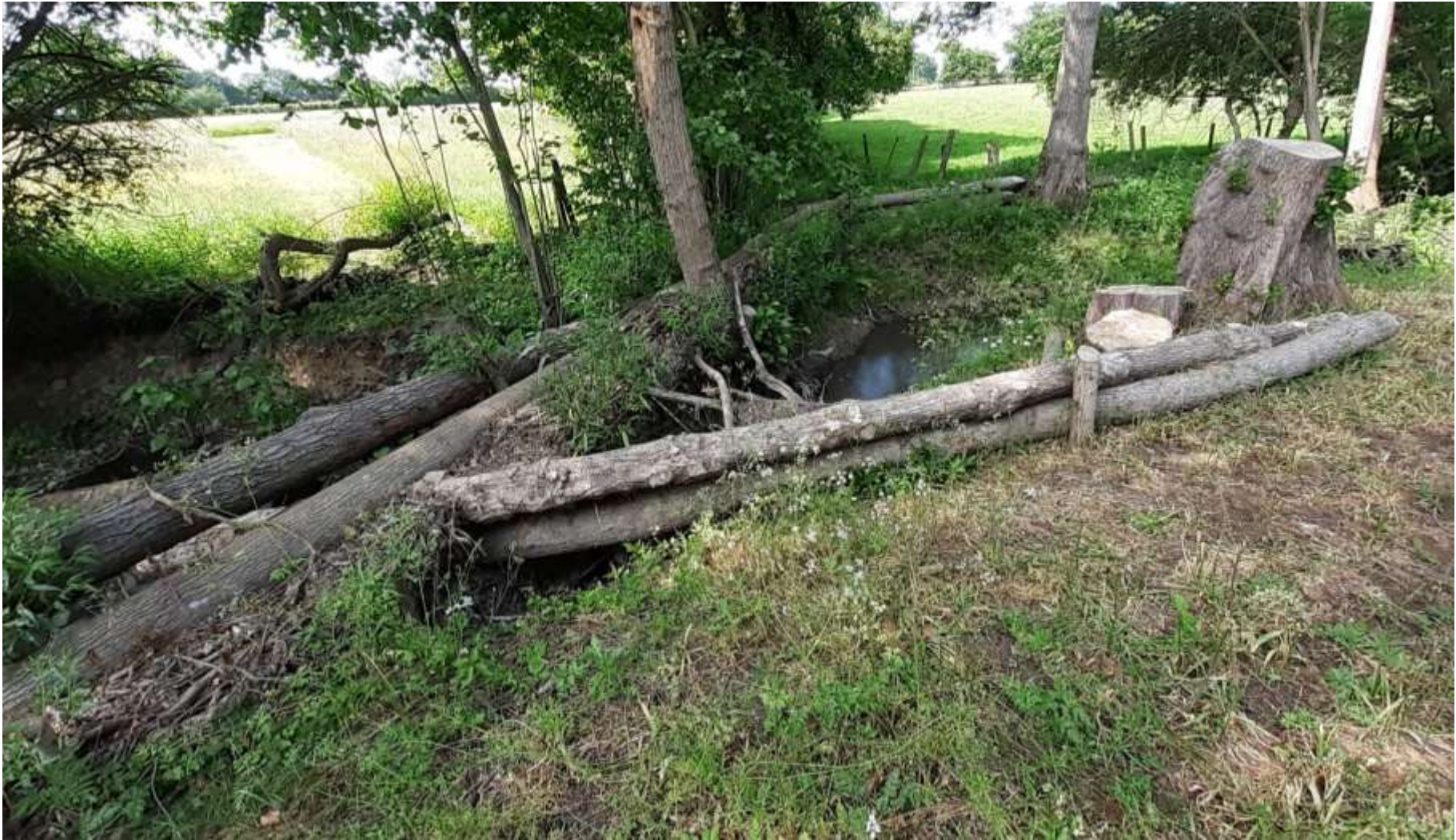
Photo 19 1b.1; 2b; 3b.1 Represents an example of what has been constructed at other sites using NFM principles. As stressed in the specification, it will depend on the character of the watercourse, what we want the dam to achieve, and the contractor's creativity and capability.
