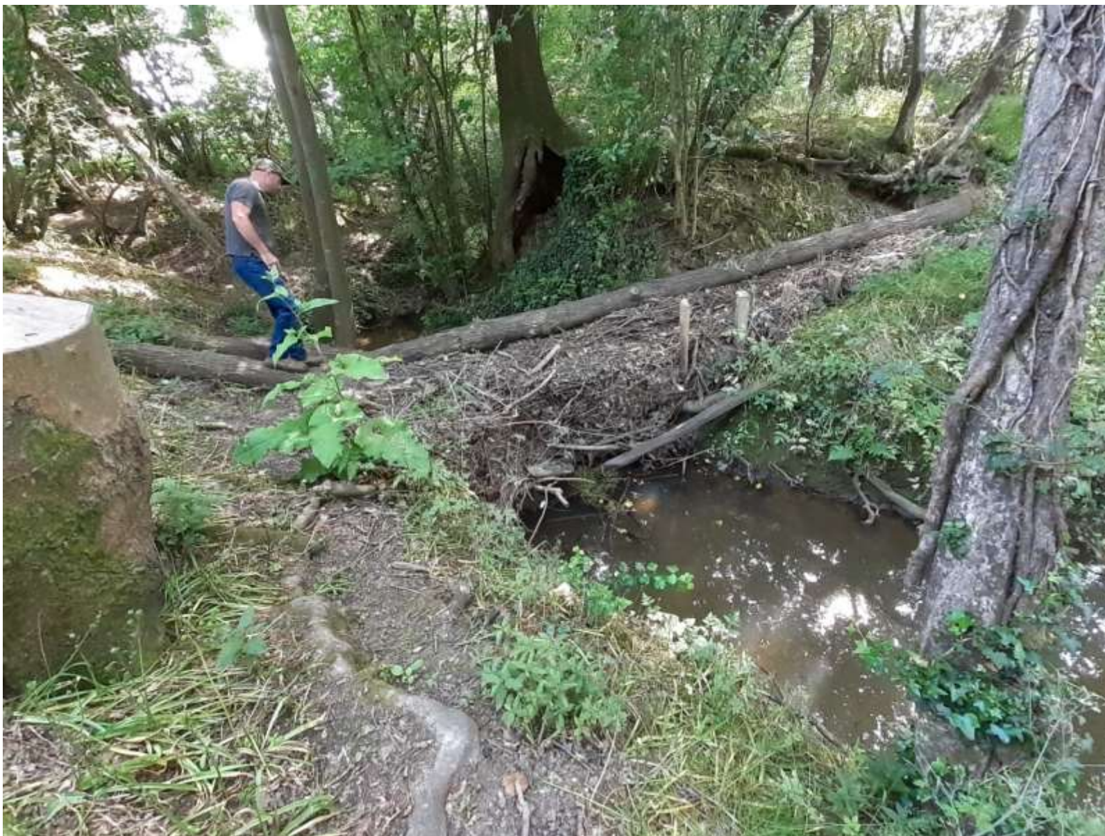
Photo 22 1c Example of what a 'meander dam' may look like when complete, with a layer of faggot bundles in front and larger trees embedded into the bank and felled on top to keep in place in high flood events
