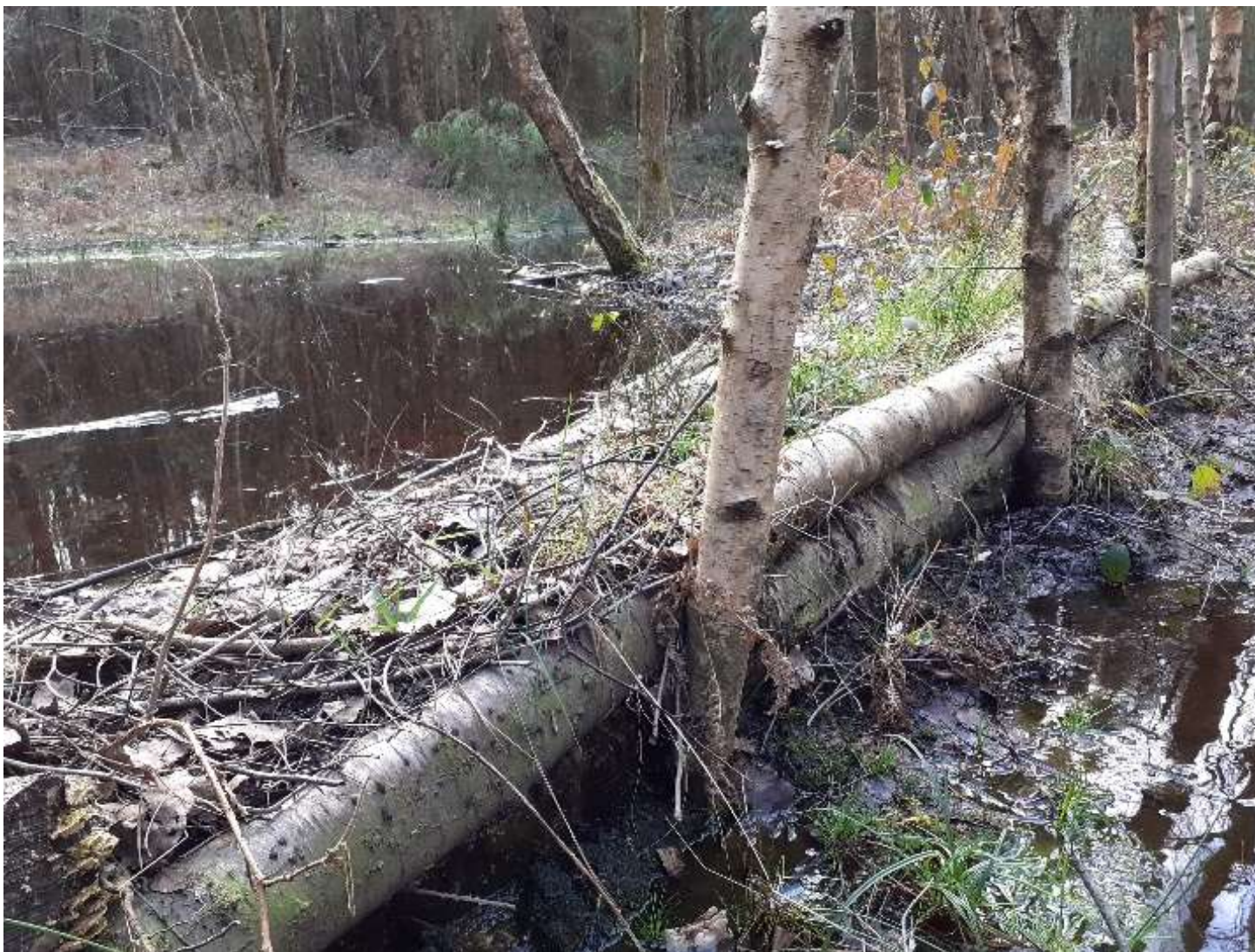
Photo 15 1b.1; 2b; 3b.1 Represents an example of what has been constructed at other sites using NFM principles. As stressed in the specification, it will depend on the character of the watercourse, what we want the dam to achieve, and the contractor's creativity and capability.
