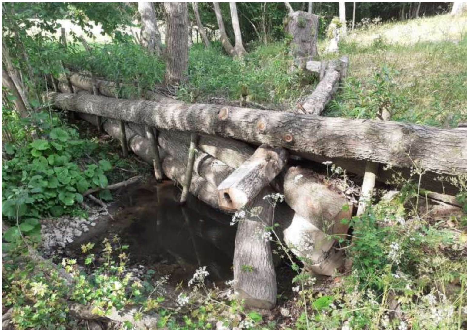
Photo 20 1b.1; 2b; 3b.1 Represents an example of what has been constructed at other sites using NFM principles. As stressed in the specification, it will depend on the character of the watercourse, what we want the dam to achieve, and the contractor's creativity and capability.
