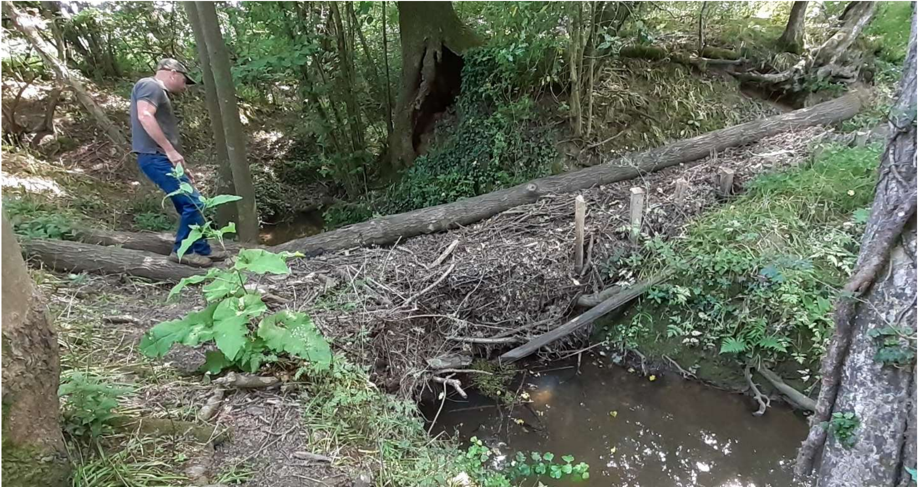
Photo 18 1b.1; 2b; 3b.1 Represents an example of what has been constructed at other sites using NFM principles. As stressed in the specification, it will depend on the character of the watercourse, what we want the dam to achieve, and the contractor's creativity and capability.
