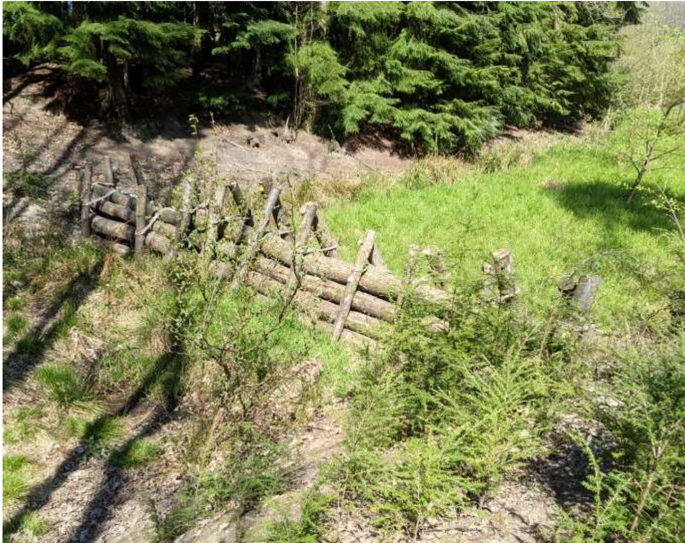
Photo 16 1b.1; 2b; 3b.1 Represents an example of what has been constructed at other sites using NFM principles. As stressed in the specification, it will depend on the character of the watercourse, what we want the dam to achieve, and the contractor's creativity and capability.
