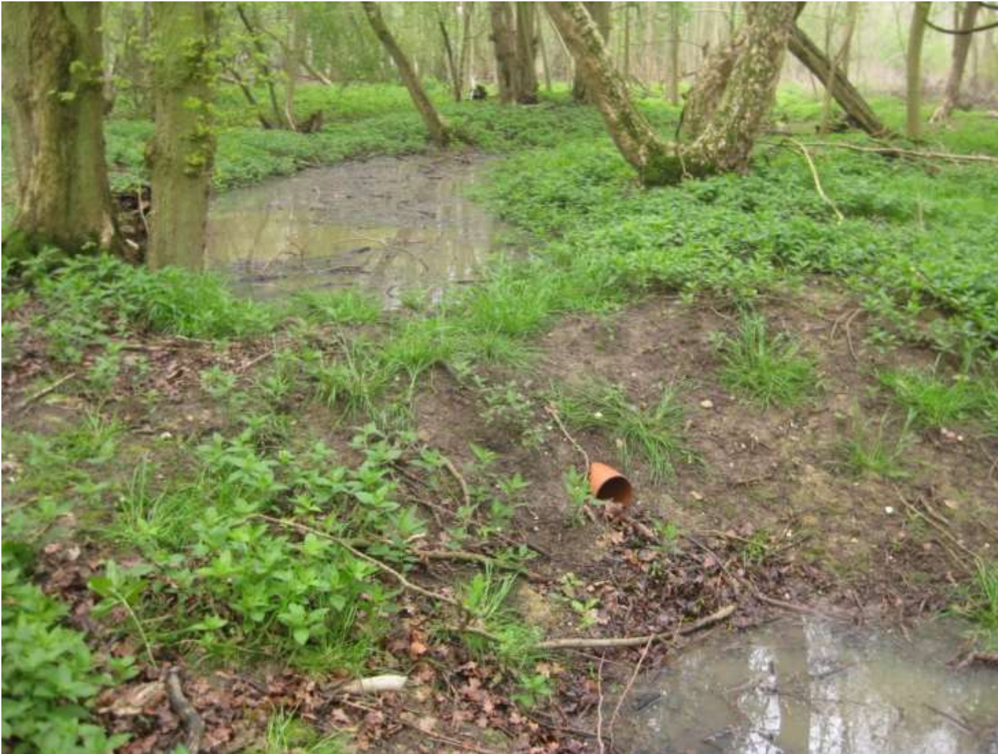
Photo 21 1b.2 Example of earth dam made for water retention at an RSPB site. Earth dams at RSPB will have a larger crest and lower pipe with elbow attachment, but the size and overall nature of the structure is similar.
