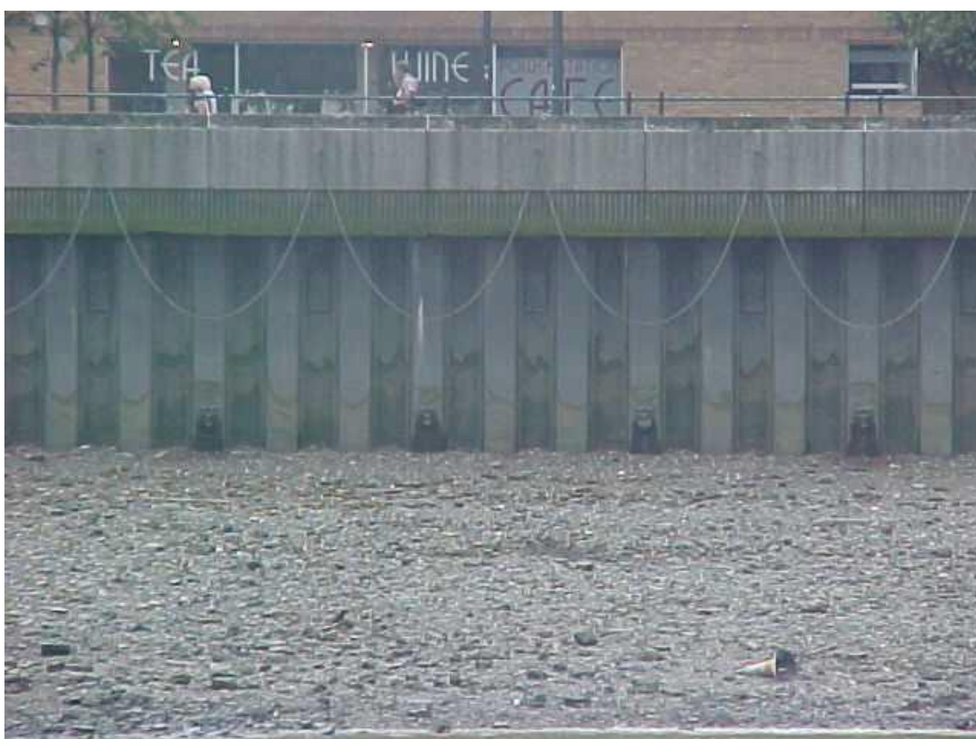
Type: Sheet Piling
