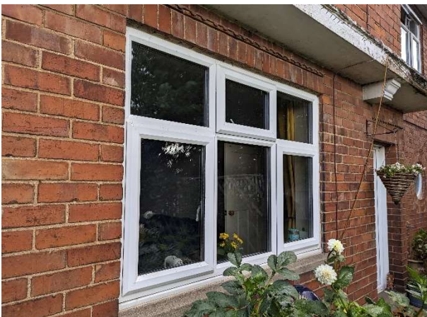
Photo 3 – Overview of uPVC double glazed window units.
