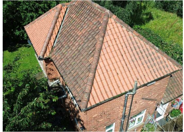
Photo 26 – Overview of the roof.
