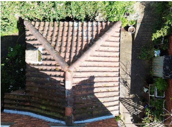
Photo 29 – Overview of clay tiles over 1 storey extension.
