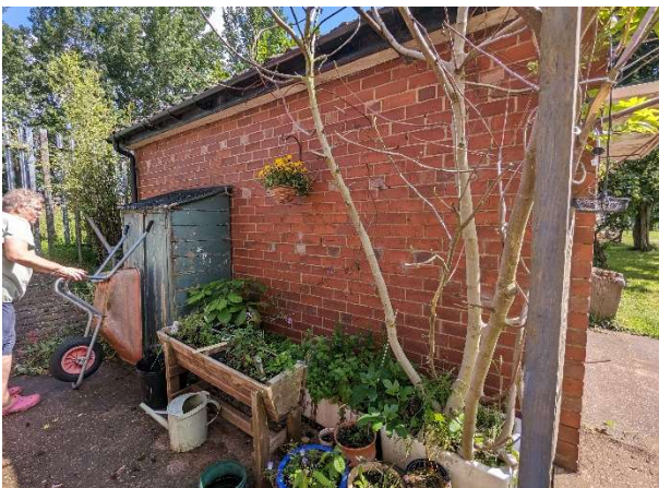
Photo 23 – Overview of brickwork for the Garage.
