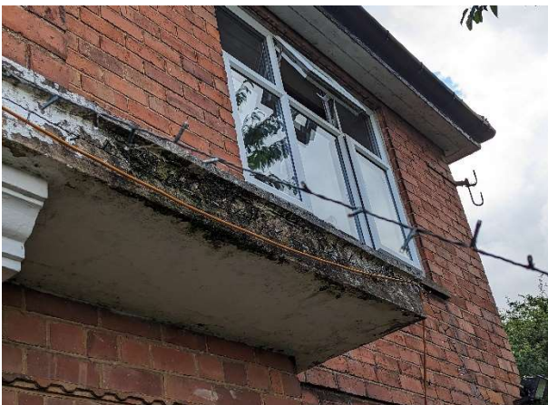
Photo 5 – Concrete canopy over main front entrance on the southern elevation.
