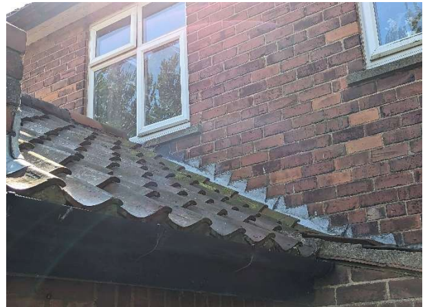
Photo 14 – Overview of the clay tiles and flashings.
