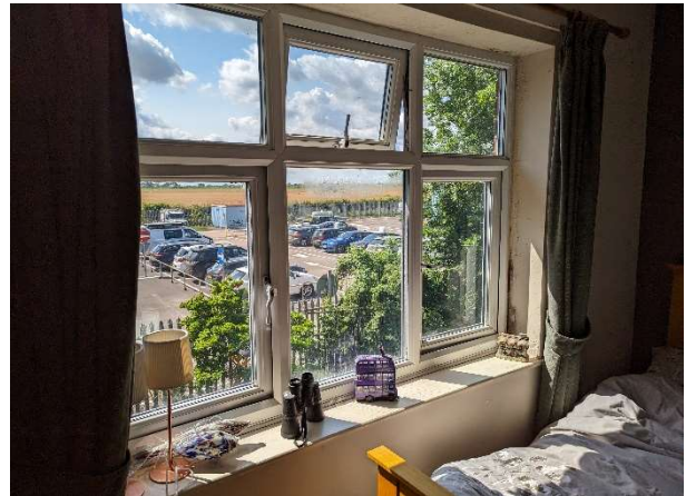
Photo 50 – Overview of the window to Bedroom 2.
