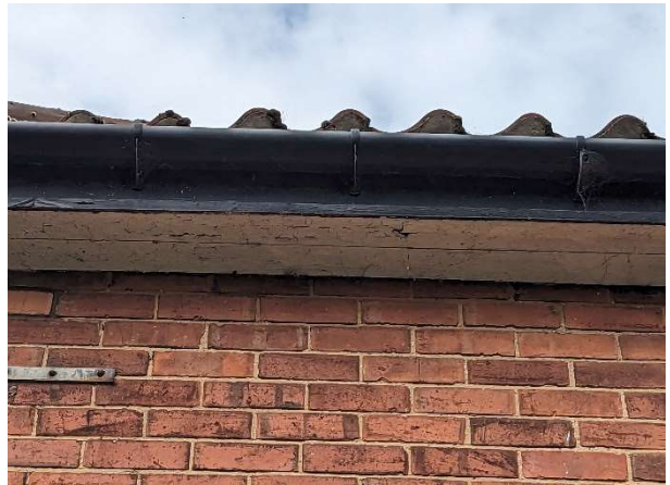
Photo 20 – Overview of timber soffit/fascia.
