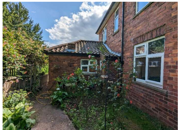
Photo 12 – Overview of 1 storey extension on the northern elevation.
