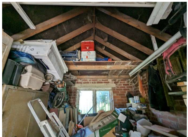
Photo 22 – Internal view of Garage.
