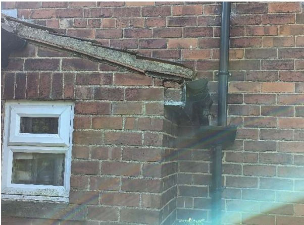
Photo 13 – Closer view of tiles and brickwork on the northern elevation.
