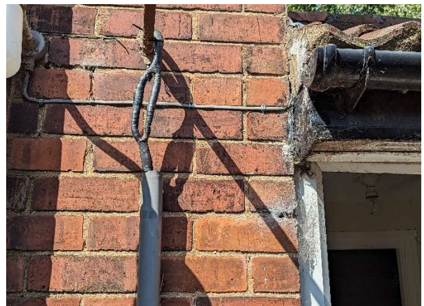
Photo 18 – Closer view of condition of brickwork.
