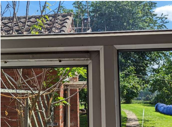
Photo 43 – Trickle vent installed to Kitchen window.
