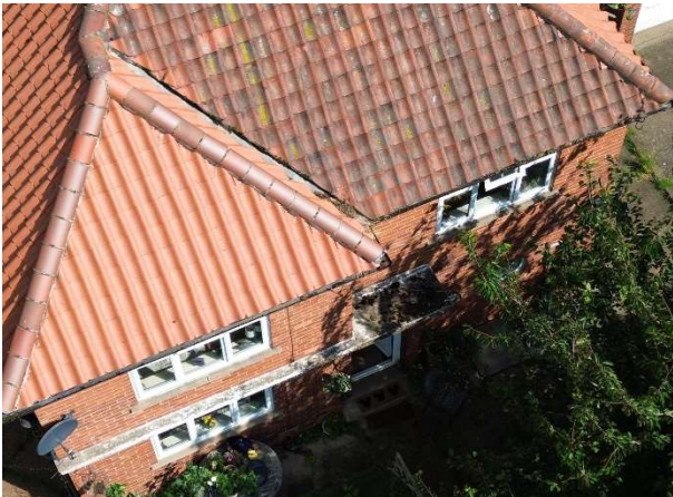
Photo 31 – Overview of the roof.
