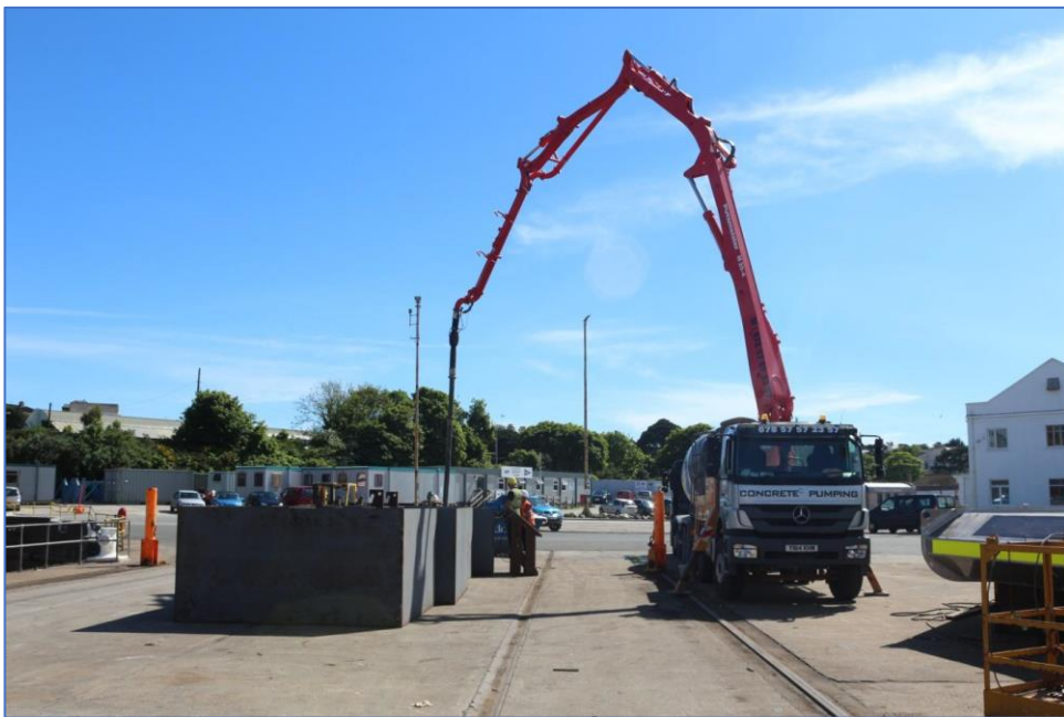
Figure 3 - Construction of Square Ancillary Clumps
