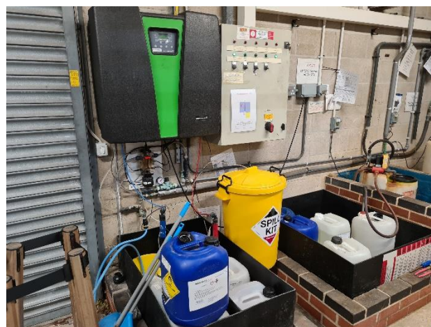
MCW Inlet 1 & Chlorine dioxide unit – Plant room
