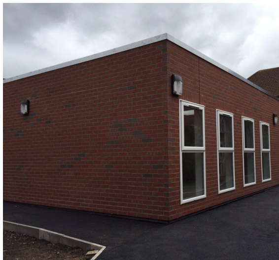
Example of brick slip cladding to a modular building
