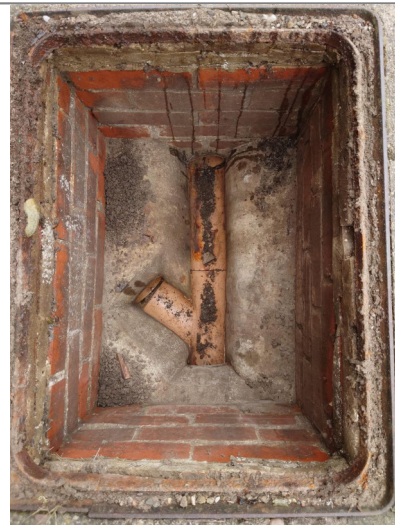
Manhole / Access Point: MH1 Internal
