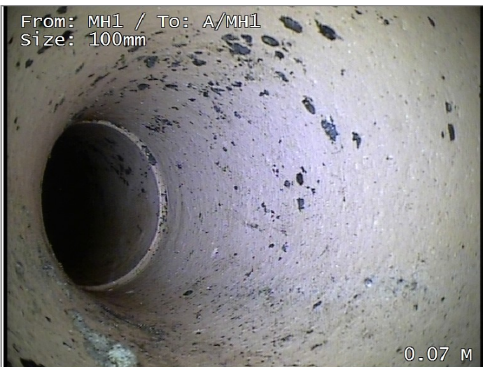
Line of drain/sewer deviates left
