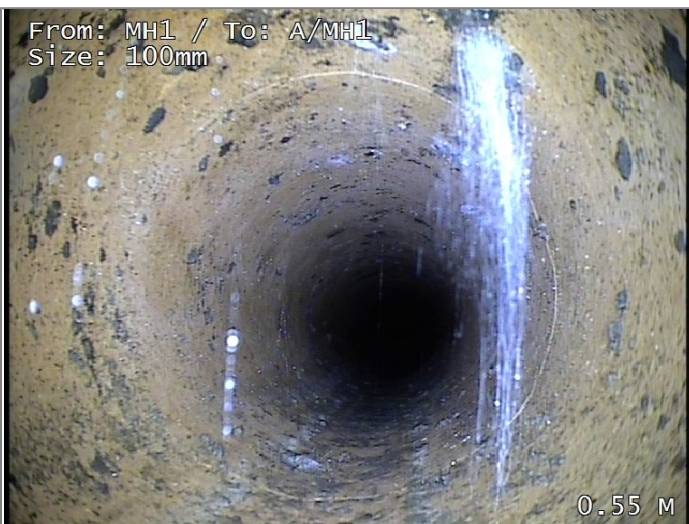
Crack circumferential from 6 to 6 o'clock
