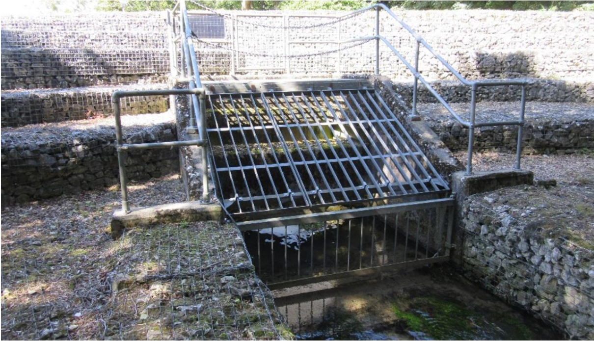
Figure 2-5: Downstream culvert outlet (photo taken August 2019)
