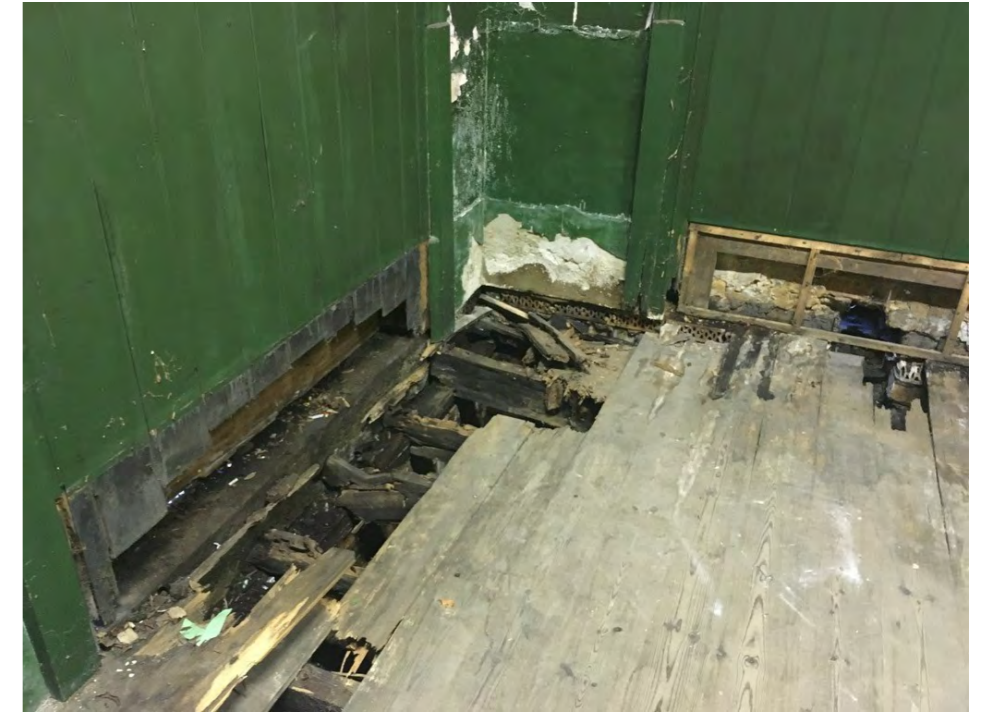
Plate 20: Water damage present within the 'Booking Office'
